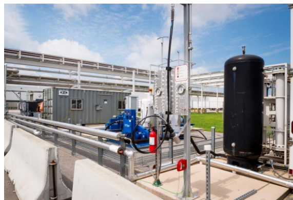
“First ever” fueling of fuel cell product (MHE) of hydrogen reformed from landfill gas. Testing showed no difference in stack performance vs. delivered H 2 source.
