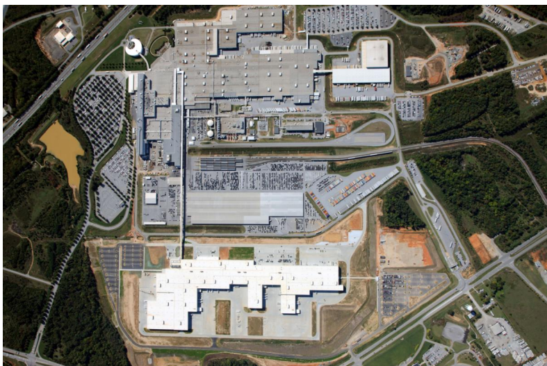
BMW South Carolina assembly plant: world's largest fuel cell deployment at one site.
