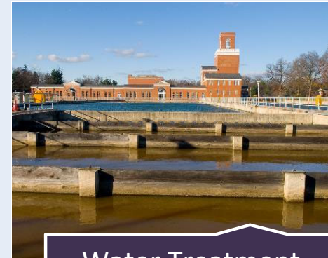
Water Treatment and Infrastructure
