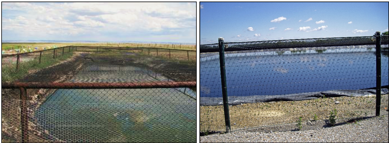
Figure 4-2: Pits with Fencing and Netting.
