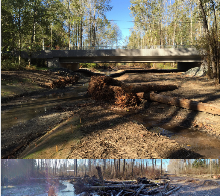
Estuary Project - Bellingham, Washington Squalicum Creek Reroute
