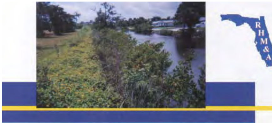
Figure 191: Stepped GeoWeb shoreline, Vero Beach Florida 1994. Source: R.H. Moore & Associates, Inc.
