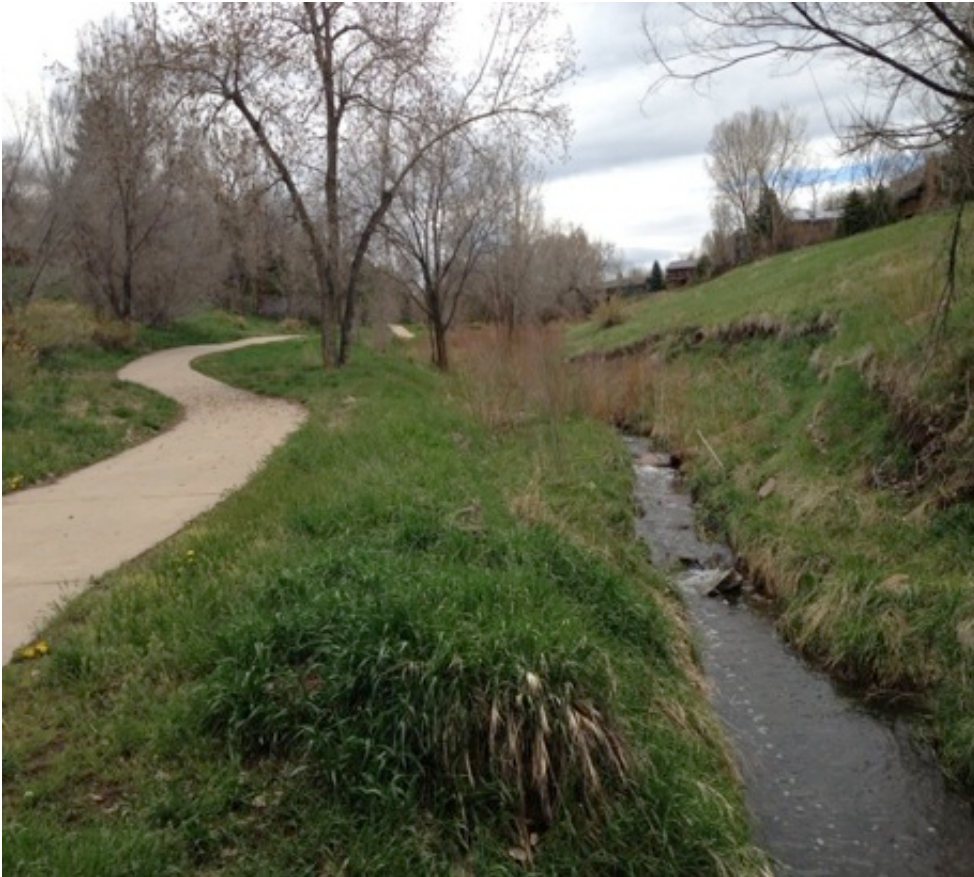
Stormwater in Tucker Gulch. Golden, CO
