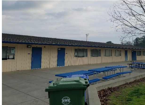
Sacramento region high school (7 portable classrooms)
