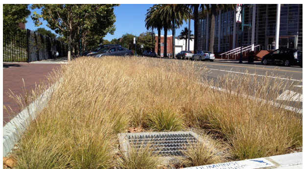
A "green street" uses practices such as porous pavement and bioretention to capture, infiltrate, and evapotranspire stormwater, preventing contaminated runoff from reaching local waterbodies.
