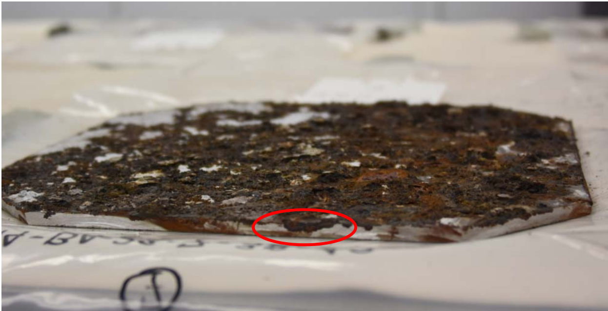
Figure A-1. Image provided by Robert Jamond on 3/20/19. This image was taken of the edge of Coupon #7 after extraction from Tank #14 and prior to shipping to IMR. The red circle identifies an area-of-concern identified prior to shipment of the coupon to IMR.
