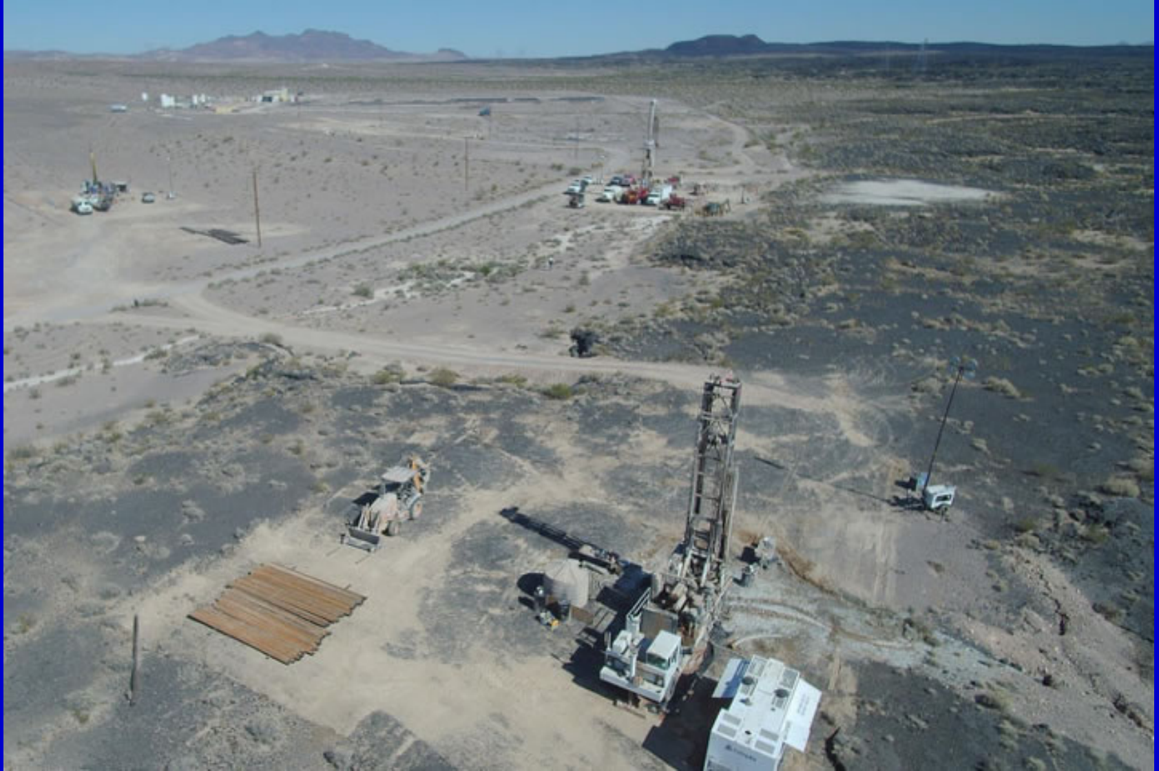
Fort Cady Site in October 2017 showing drilling activity, and pilot plant in the background.
