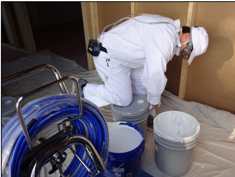
Figure 1. Opening 5-gallon Paint Buckets and Airless Sprayer Hose.
