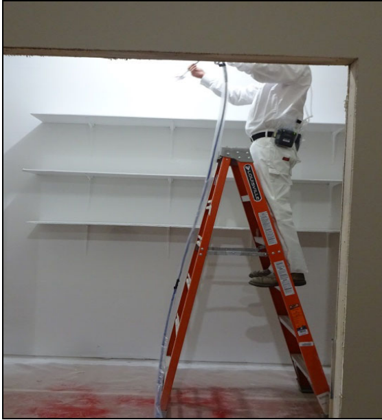
Figure 4. Spraying Above Shelving in Test Room Using a Ladder.
