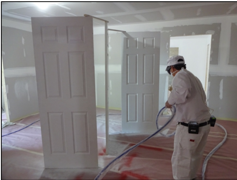
Figure 3. Spraying Doors in Test Room Built for Airless Sprayer Study.
