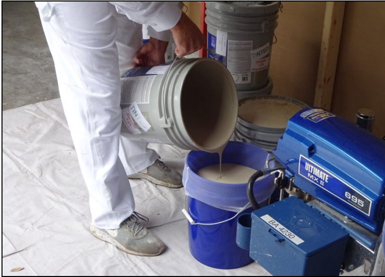
Figure 2. Pouring Paint Through Strainer (Intake Hose on Outside of Strainer Bag).
