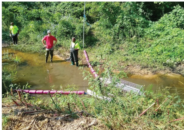
Installation of Litter Gitter on Proctor Creek.
