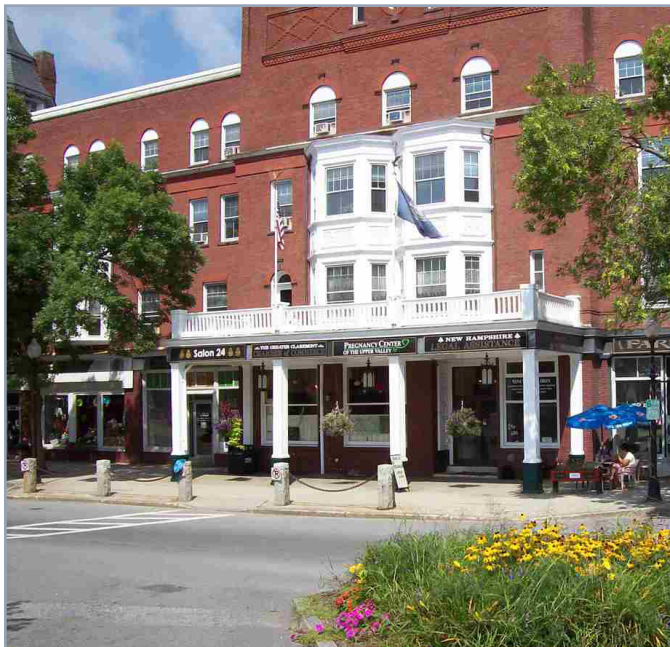
Renovated Opera House Square Building.
