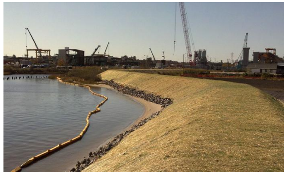
One of two berms confining dredged sediment at the Atlantic Wood Industries Superfund Site in Portsmouth, Virginia.
