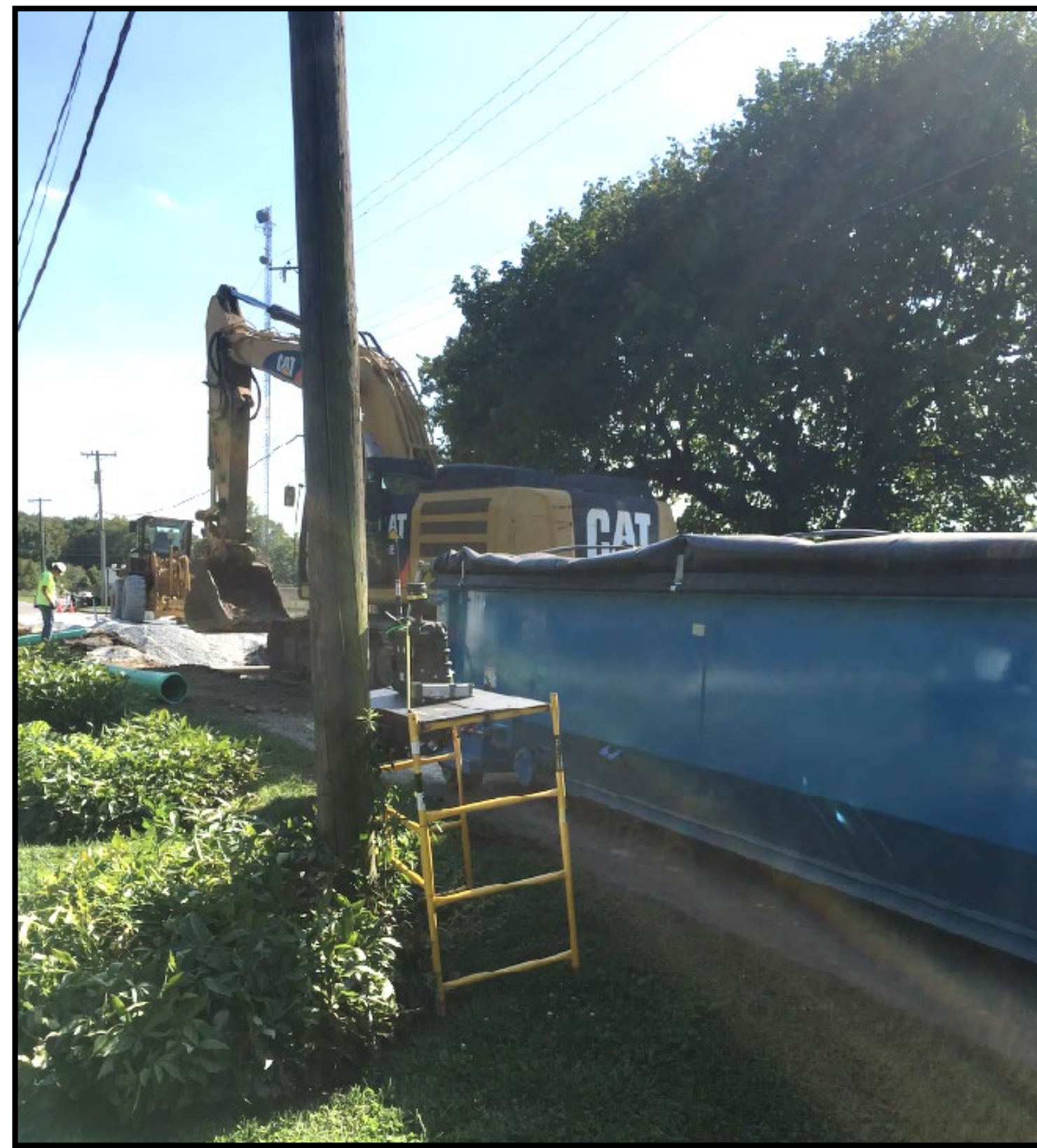
Air monitoring station
