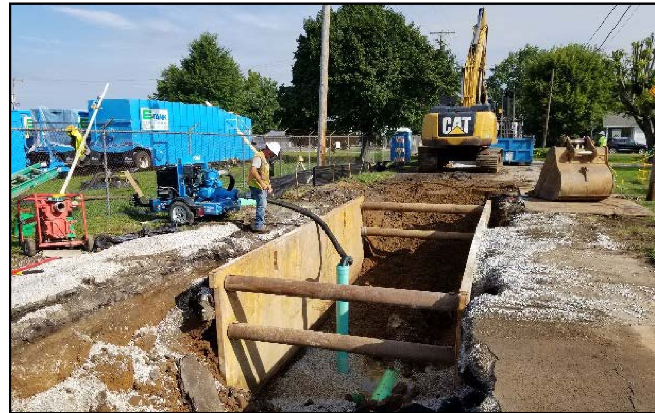
Trench for new sewer line
