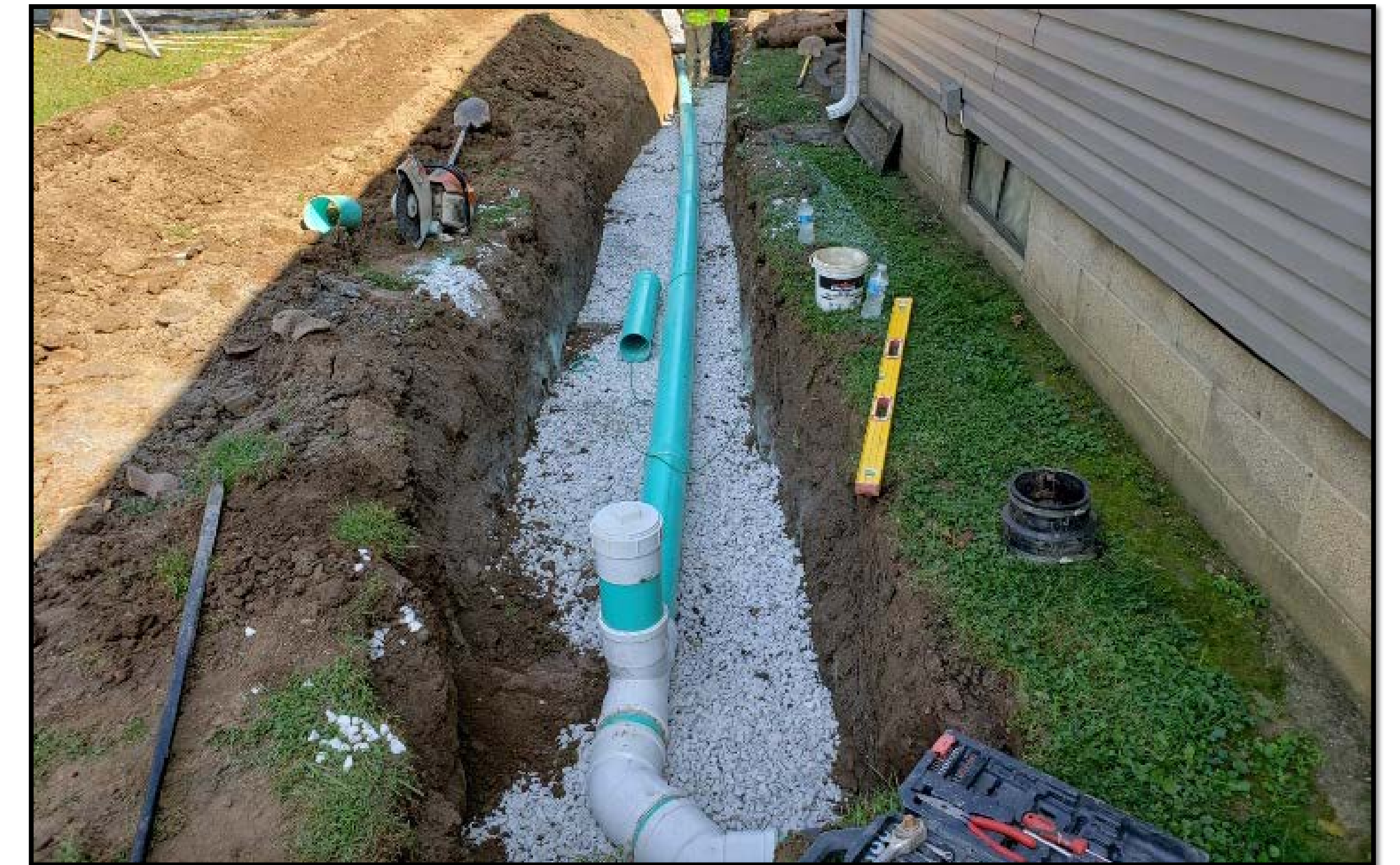
Sewer connection pipe replacement at home
