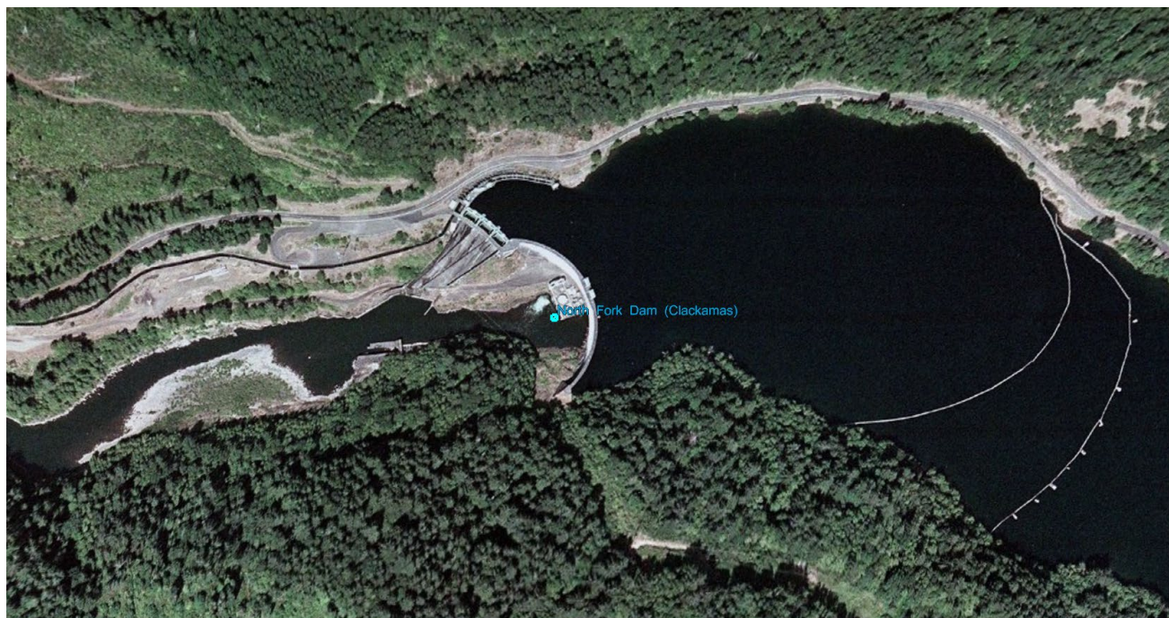
Figure 9-2. PGE's North Fork Dam and Reservoir on the Clackamas River.
