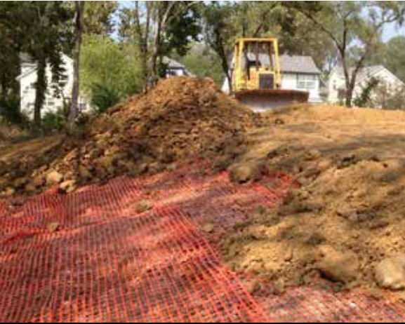
The construction team built a demarcation barrier to prevent digging in areas where contaminated soil couldn't be removed.
