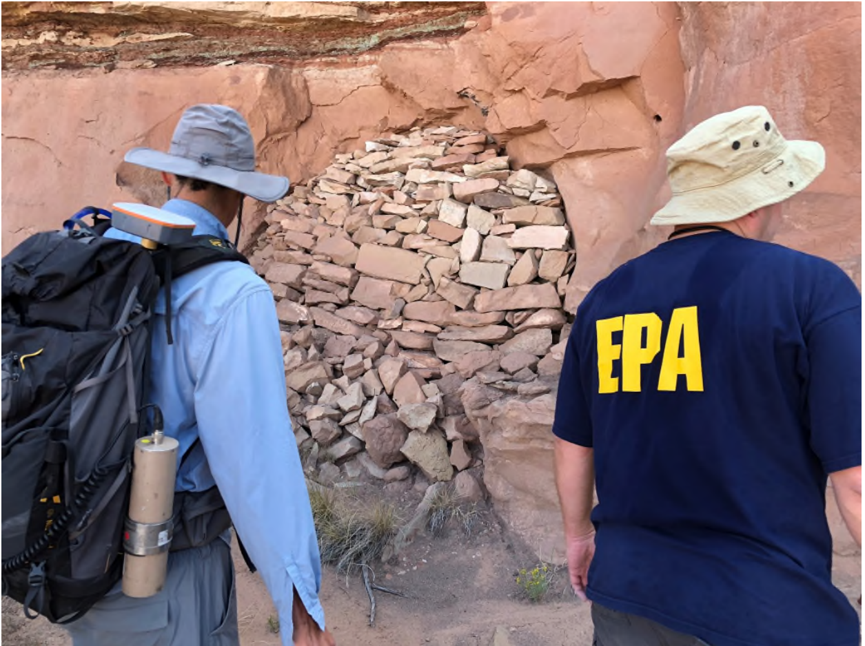
Photograph 7. EPA and Tetra Tech at a closed portal at Step Mesa.
