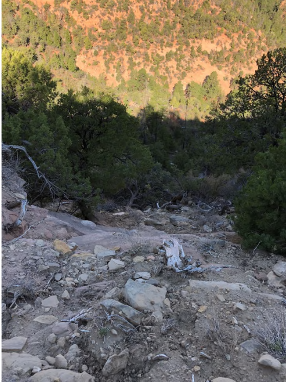
Photograph 13. Extreme Slope at Western Waste Piles of Mesa IV West Mine No. 2
