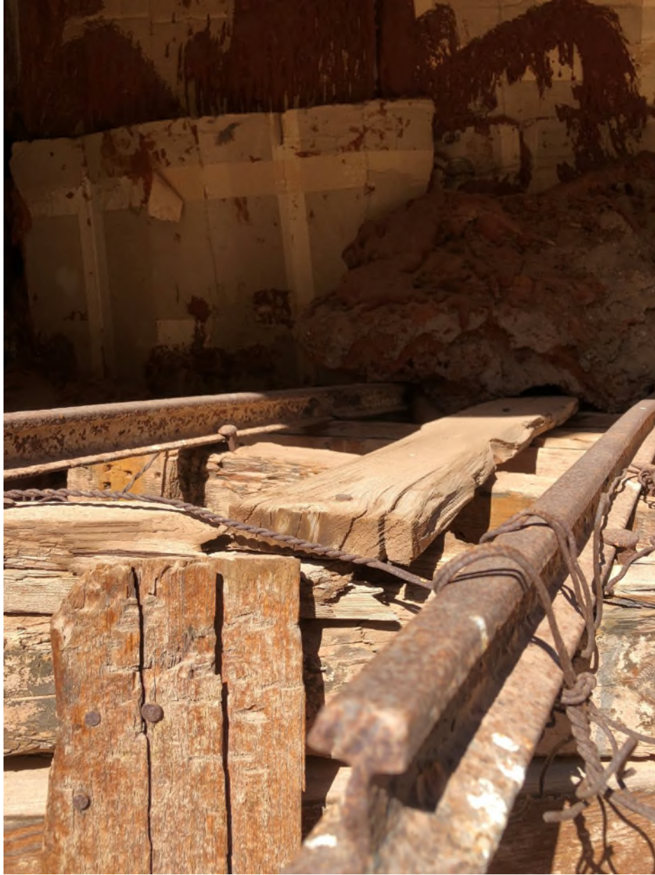
Photograph 10. Previously Reclaimed Portal at Mesa VI Mine
