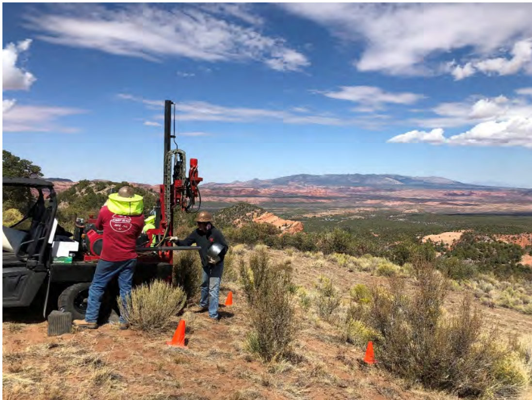
Figure 19. The Track-Mounted Drill Rig
