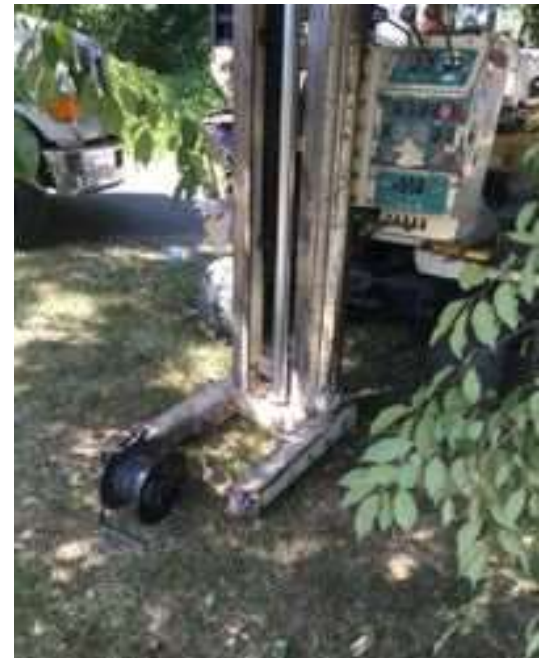
Direct-push technology used to install temporary ground water monitoring well.
