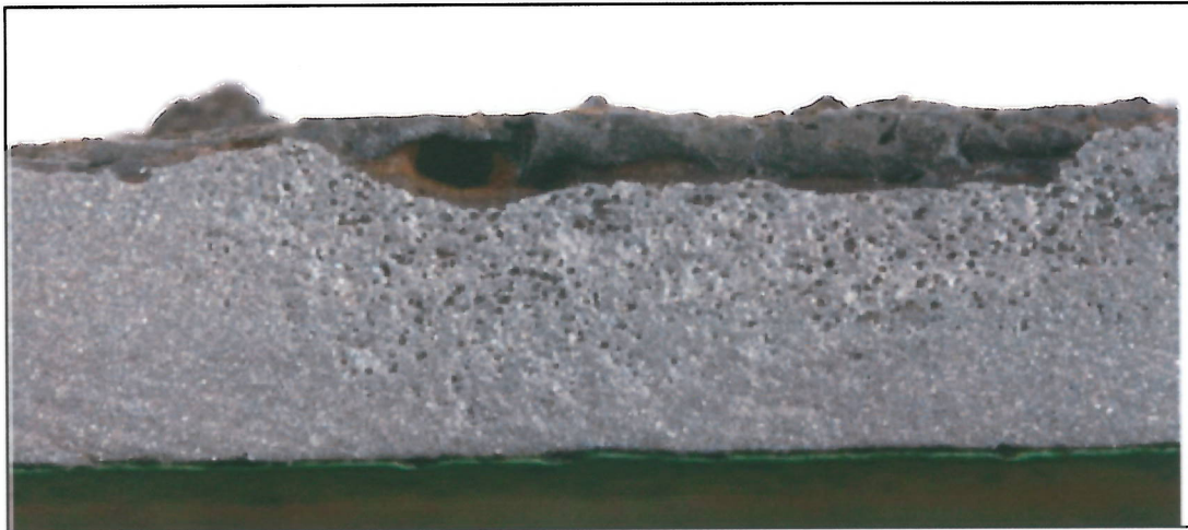
Figure A-4. Detail of the sandblasted edge on 3/20/19 in the same location as shown in the picture below. The sandblasting revealed that the feature was not a corrosion pit, as shiny metal was revealed when the red-colored staining was removed. There was an unusual appearance to the edge in this location, as though the sectioned edge had been superficially altered by heat associated with sectioning or some other post-sectioning reaction (atmospheric corrosion or corrosive media attack). That alteration gave the appearance of a deep corrosion pit.
