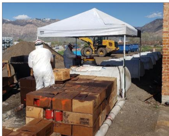
Preparing for shipment to recycling facility
