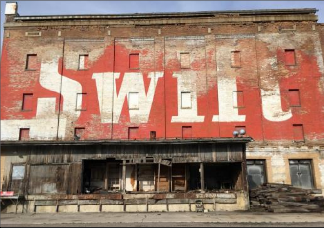
Exterior of Ogden Swift Building
