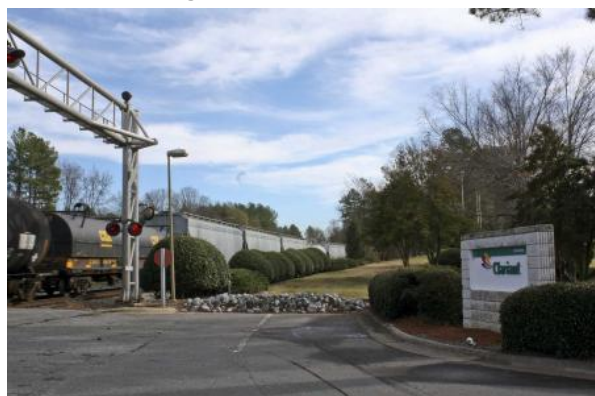
Figure 2: Rail Access at Martin-Marietta, Sodyeco Superfund Site
