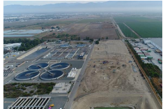
Recycling Plant No. 5 Expansion Project
