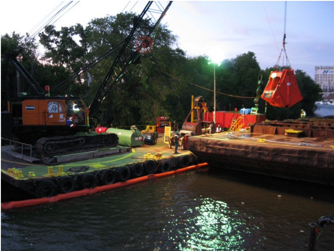
Monday, June 1 - First Bucket of Sediment Being Dredged
