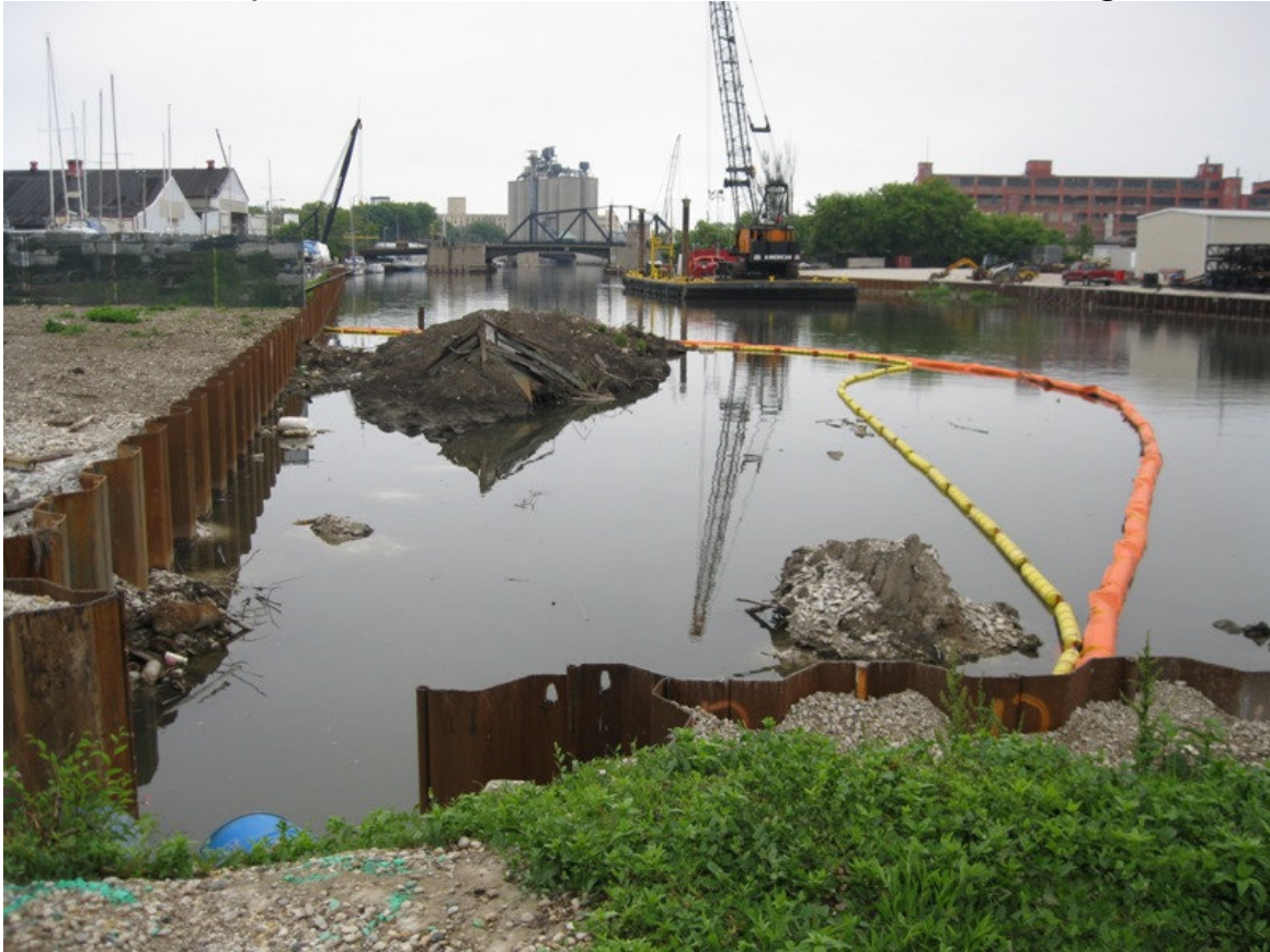
Wednesday, June 17 th - Oil Boom/Silt Curtain near abandoned tugboat
