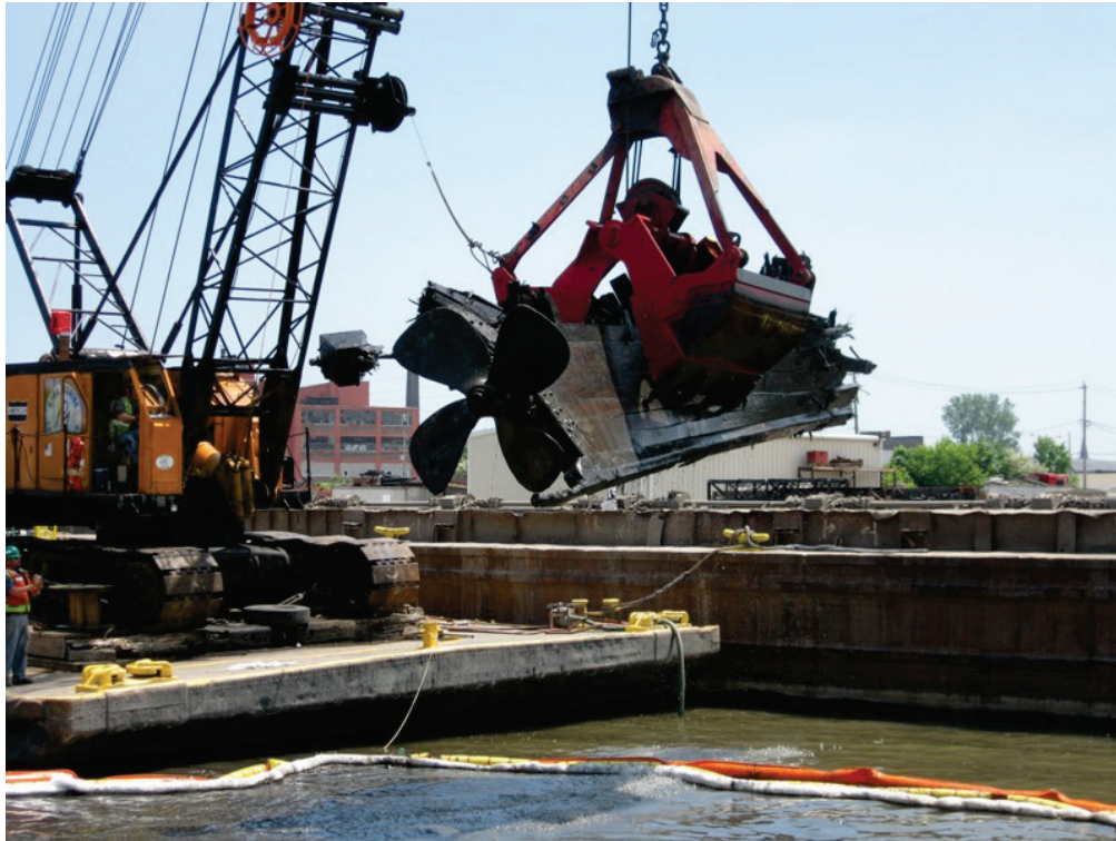
7. The propeller and driveshaft was removed in one piece.
