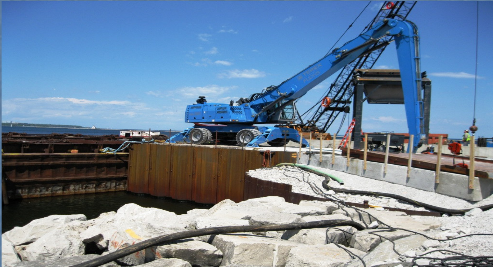
Offloading Excavator and grizzly screen being assembled at the CDF
