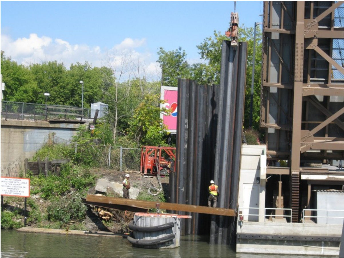
Gillen driving sheet pile at Parcel 424
