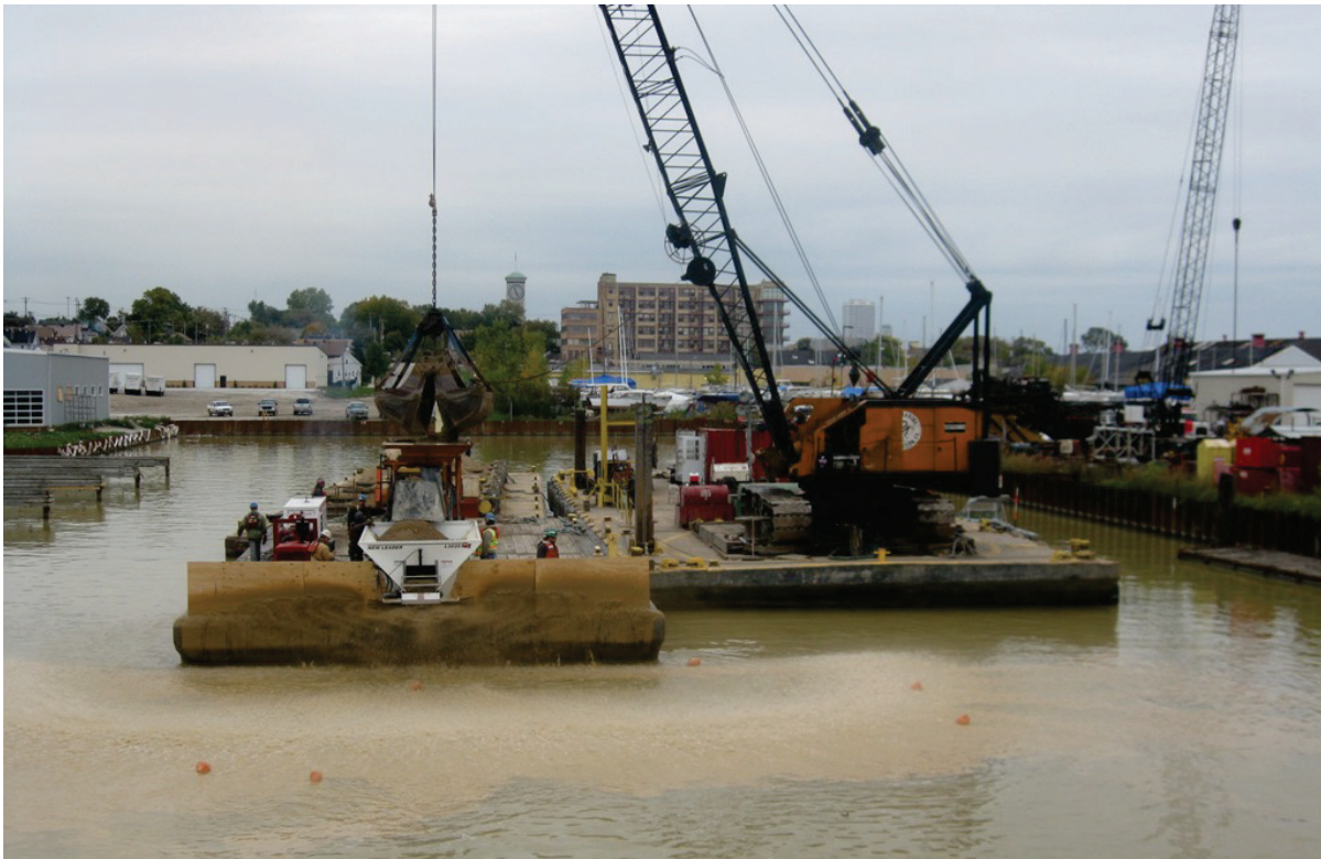
12. This is Ryba's specially designed sand spreader for thinner areas (6 to 12 inches).
