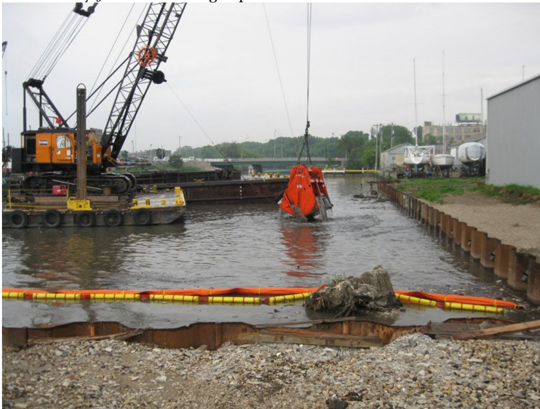
Sunday June 21 st - Dredge operations with environmental bucket.
