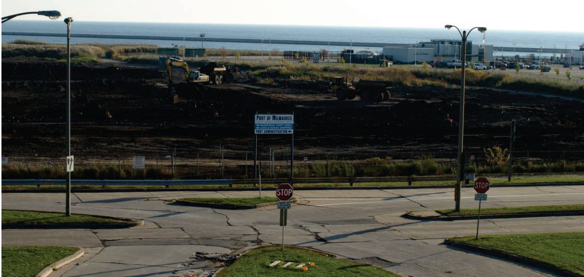
1. Freeman Environmental Services, Inc. (Freeman) and its lower-tiered subcontractor New Berlin Grading (New Berlin) constructed the cell at the CDF that contains the dredged material from the Kinnickinnic River.
