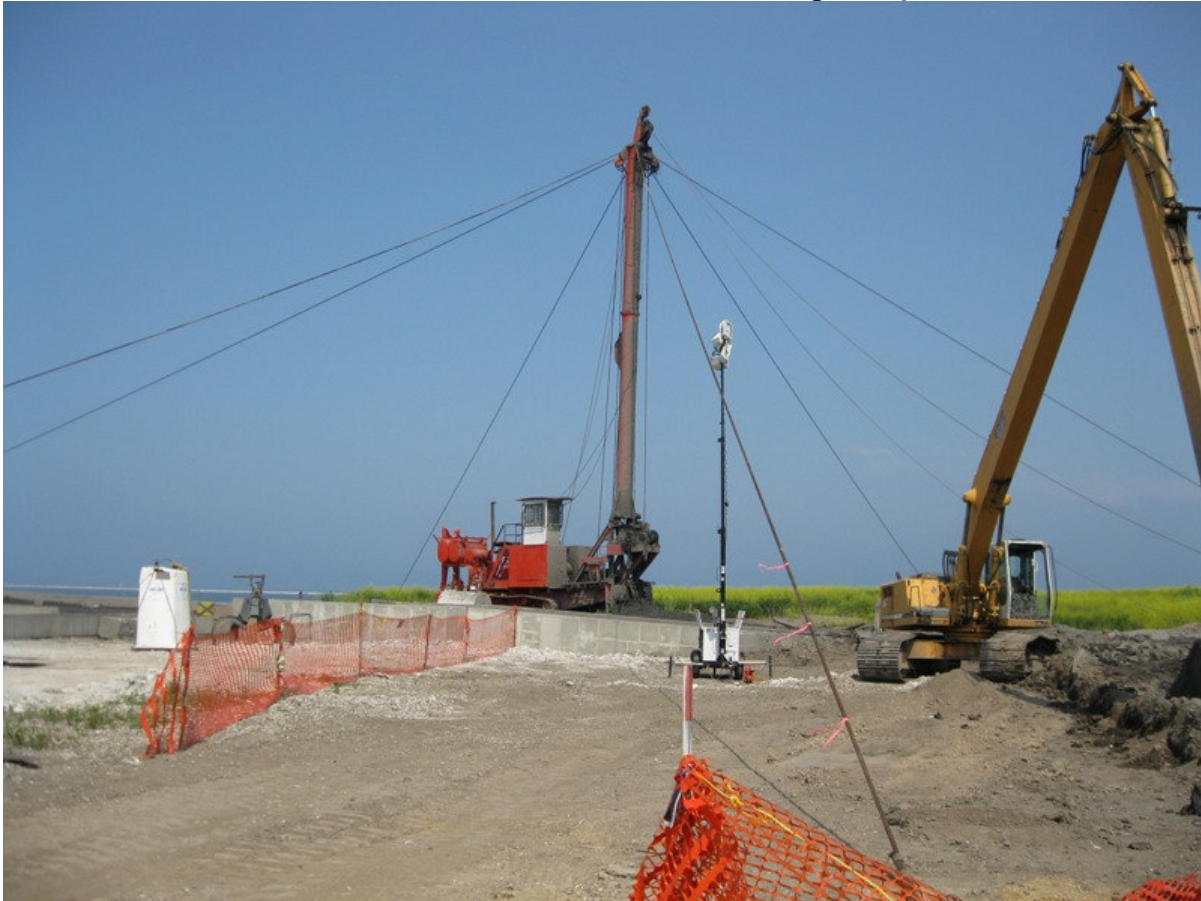
Sauerman bucket installed on dragline system
