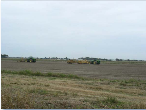
Figure 2. A farmer implements irrigation land leveling, which reshapes the land to a chosen grade and will permit uniform and efficient application of surface irrigation water without causing significant erosion.
