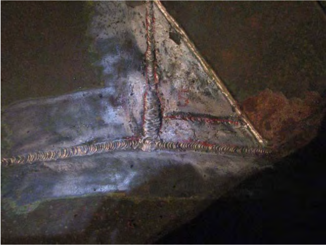
Intersecting welds between plates 4 and 5 of course 1 and the floor.
