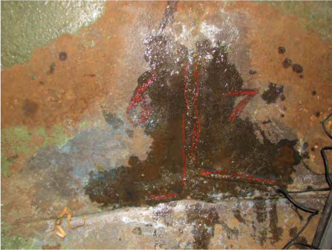
Intersecting welds between plates 6 and 7 of course 1 and the floor.
