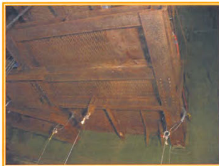
Photo #1: Cat walk framing by the tank entrance
