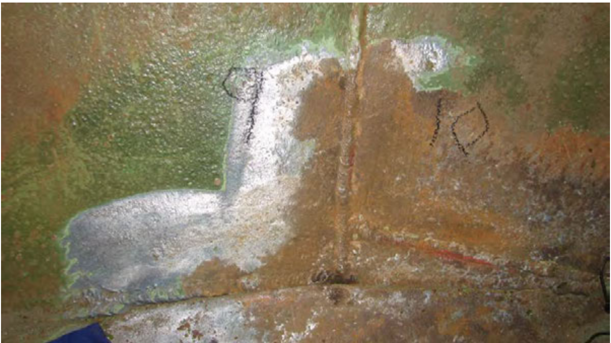
Intersecting welds between plates 9 and 10 of course 1 and the floor.
