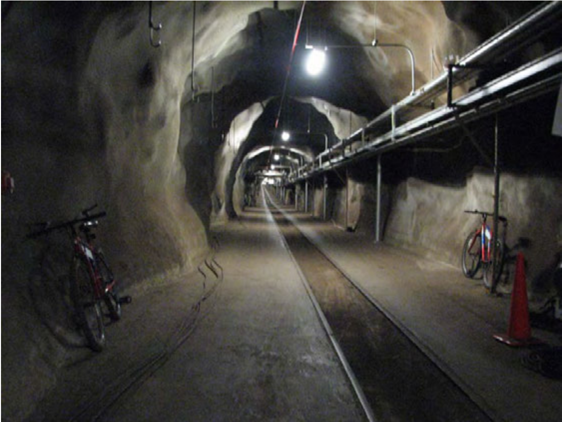
A view of the tunnel area around tank #2.
