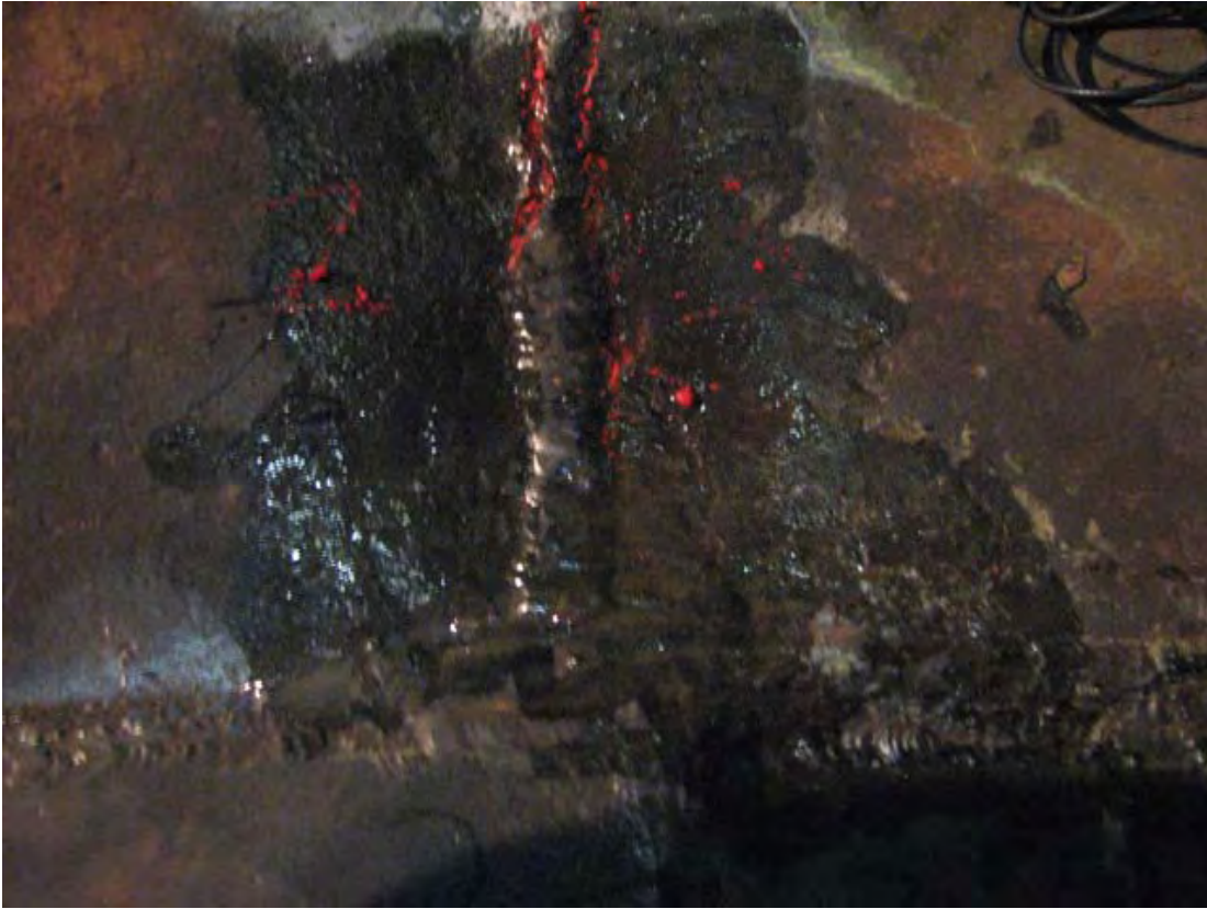
Intersecting welds between plates 2 and 3 of course 1 and the floor.
