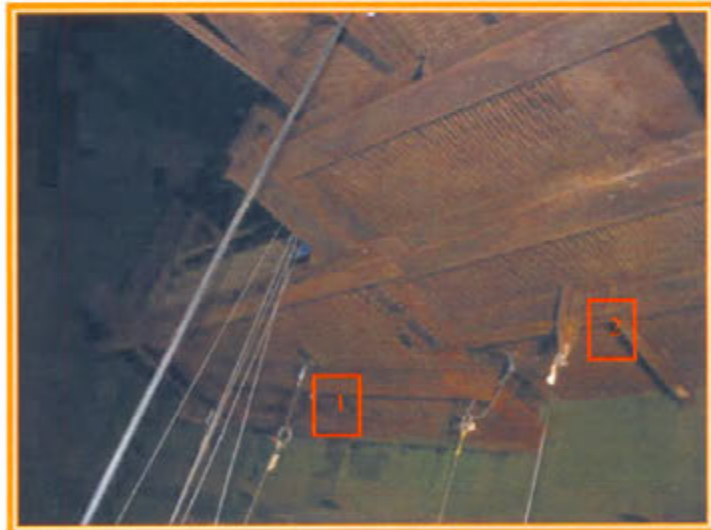
Photo #5: Proposed scaffold will be hung on points 1 & 2
