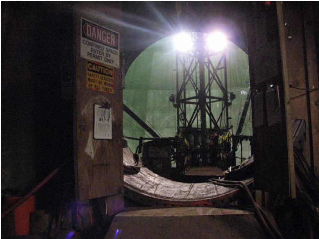
A view of the manway leading into tank #2.
