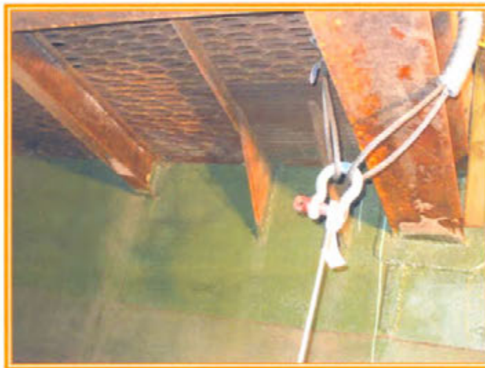
Photo #3: Weld of the major I-beam is in good condition
