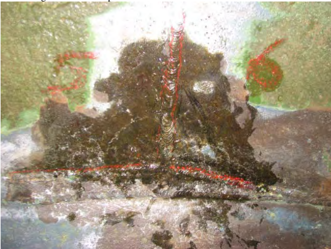
Intersecting welds between plates 5 and 6 of course 1 and the floor.
