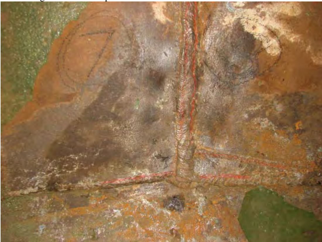
Intersecting welds between plates 7 and 8 of course 1 and the floor.
