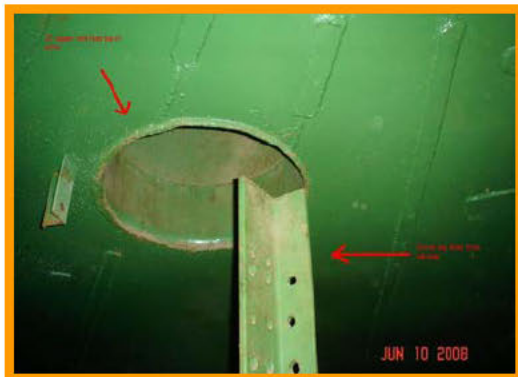
Image# 2: Showing Tank #20 Tower leg not welded to the tank.
