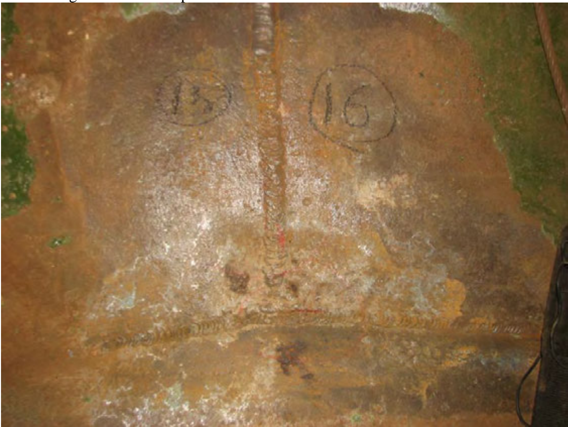
Intersecting welds between plates 15 and 16 of course 1 and the floor.
