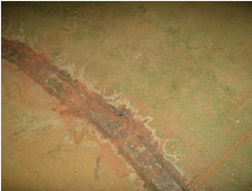
Transition from tank floor to the lower dome section
