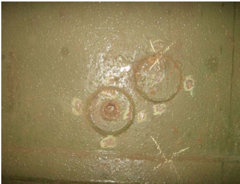
Location of piping penetration removal; Note: Condition of Coating
