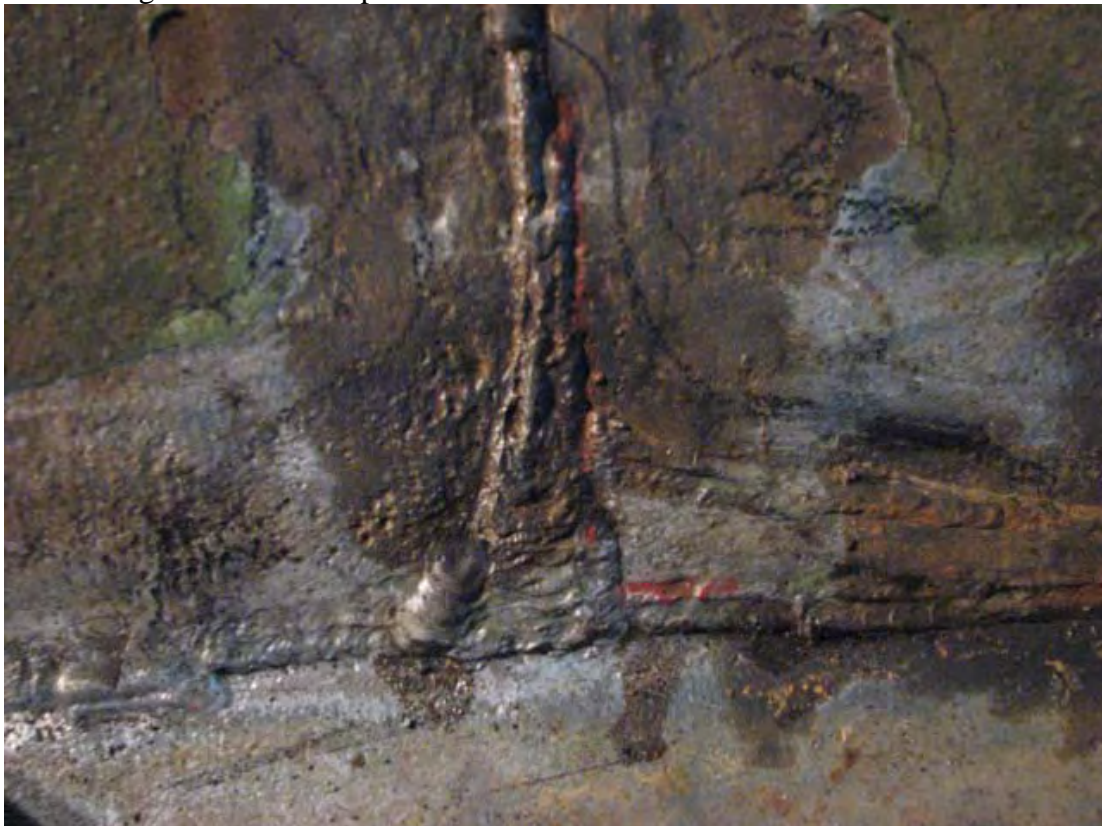
Intersecting welds between plates 1 and 2 of course 1 and the floor.
