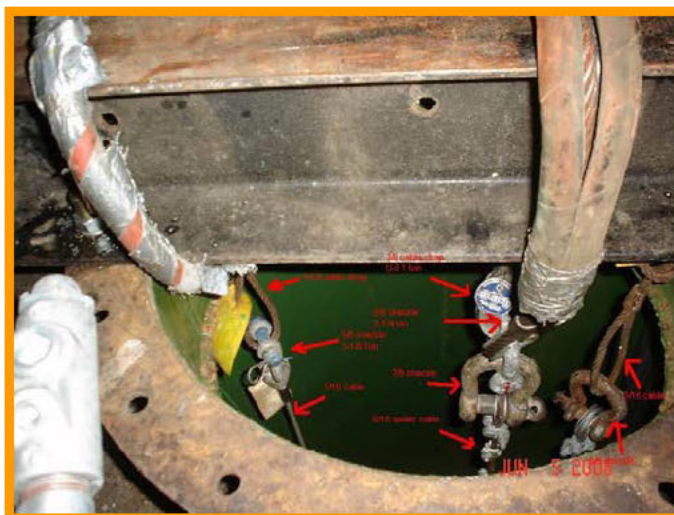
Image #4: Showing Tank #20 Spider hoist assembly cables and shackles
