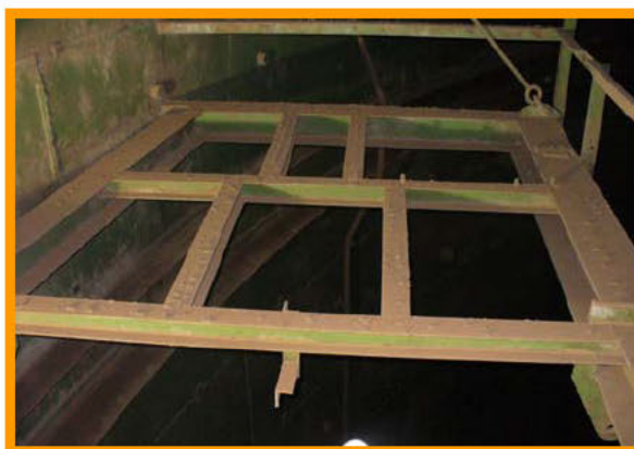
Image# 6: Showing Tank #20 Work Platform and new beam installation recommendation .
