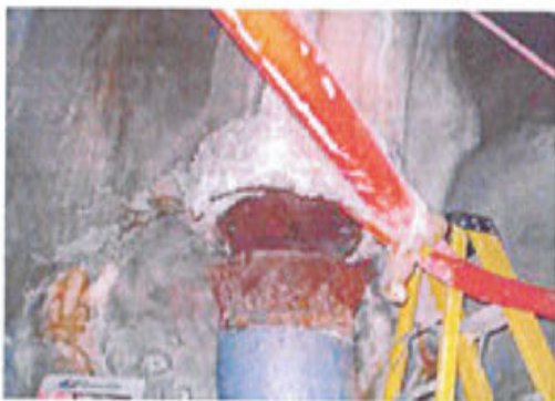
Ventilation System – Area repaired where foam was installed for ducting. Metal sheeting installed and sealed for ventilation process.
