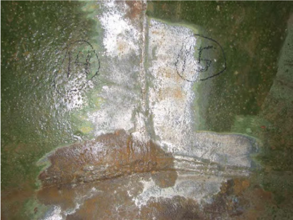
Intersecting welds between plates 14 and 15 of course 1 and the floor.
