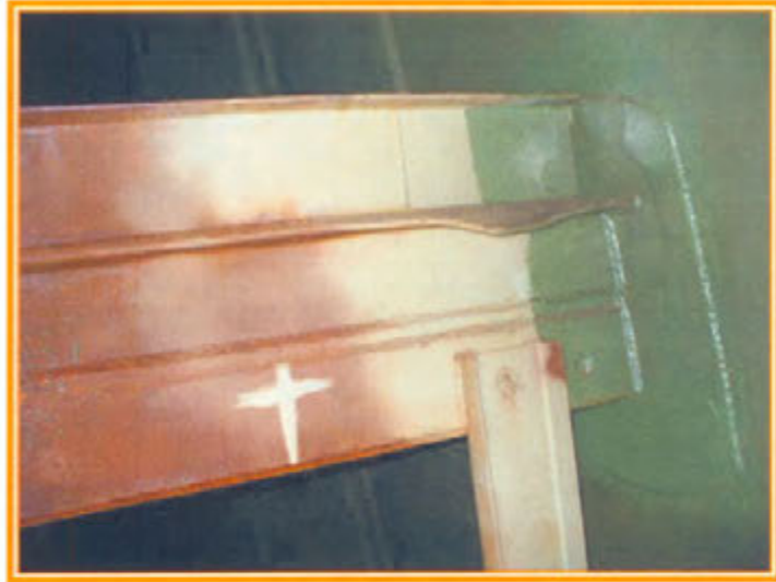
Photo #4: Weld of the major I-beam is in good condition
