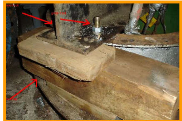
Image# 5: Showing Tank #20 Top Anchor I-Beam shortened and supported.
