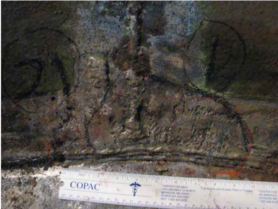
Intersecting welds between plates 21 and 1 of course 1 and the floor.
