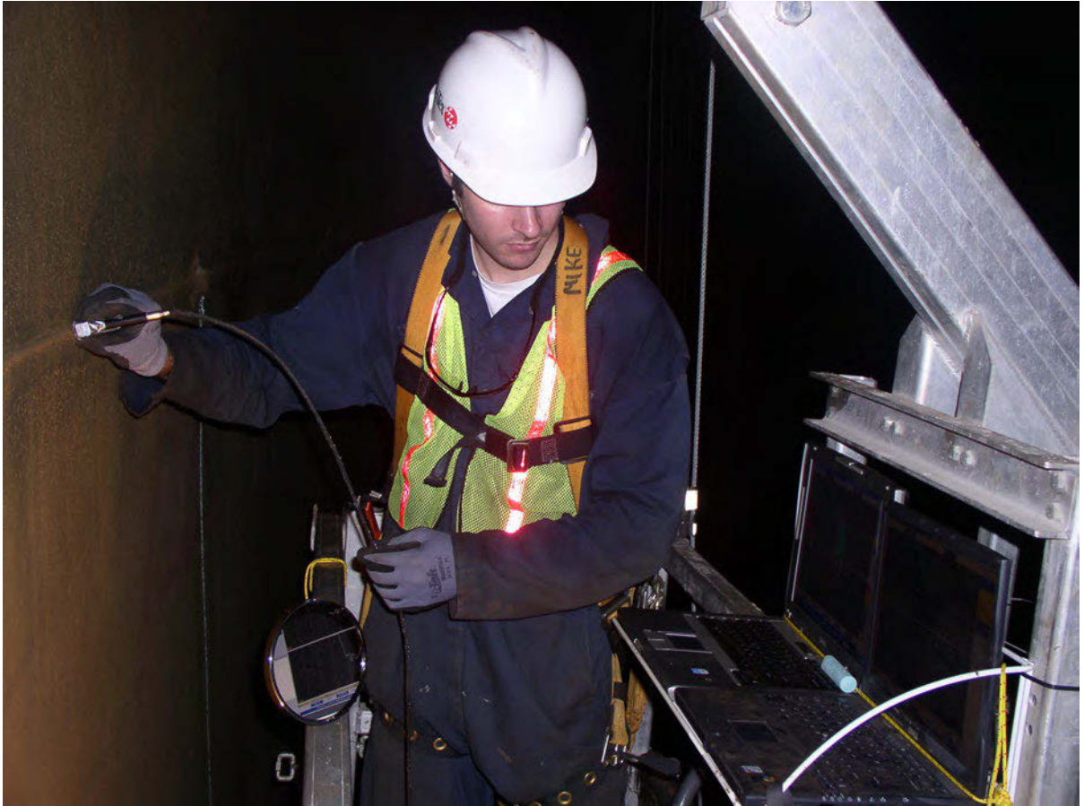
BFET (Balanced Field Electromagnetic Technique) being performed on a weld seam in Tank 6
