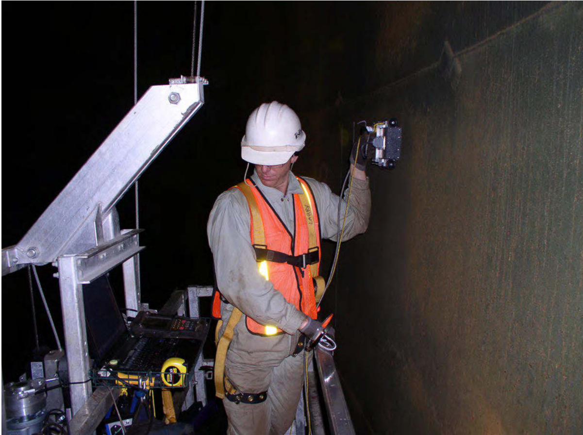
LFET scanning being performed under the catwalk on the barrel section of Tank 6
