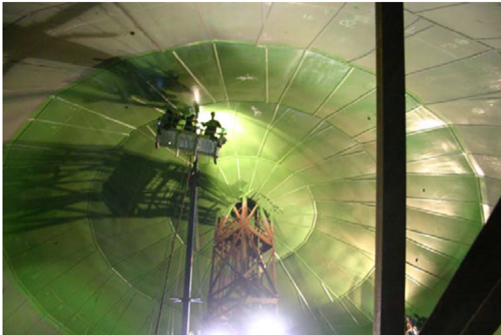
Photograph 6 – NDE technicians/examiners and operator determining the feasibility of examining course E.
