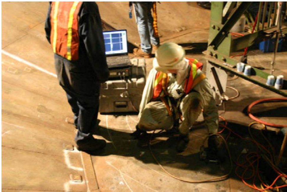
Photograph 2 – NDE technician/examiner performing LFET scanning on the tank bottom plates.
