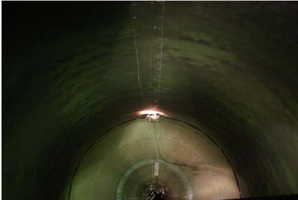
Photograph 3 – A view of the barrel and lower dome from the tower at the catwalk level.
