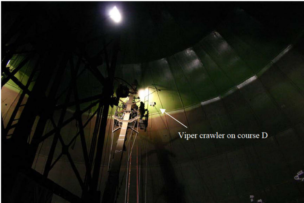
A view from the catwalk of the Viper Crawler performing an Ultrasonic Inspection of course D of the Upper Dome.
