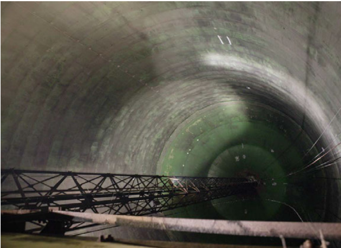
A view of tank #15 from the catwalk looking downward.
