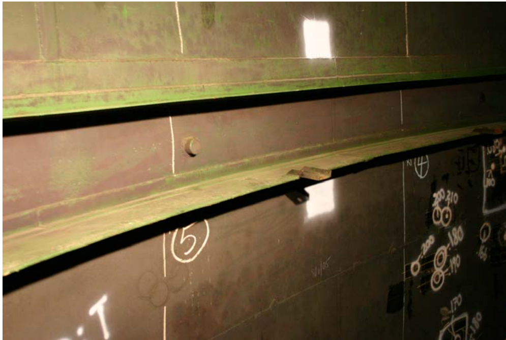
Photograph 11 – Expansion joint, quadrant B.
