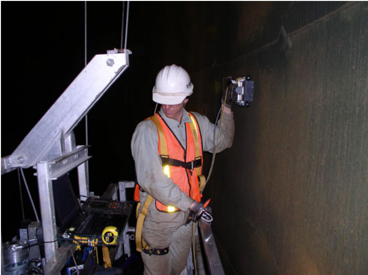
LFET scanning being performed under the catwalk on the barrel section of Tank 6
