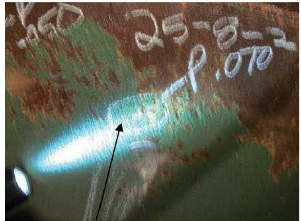
R25-P8-2 PIT REPAIR
