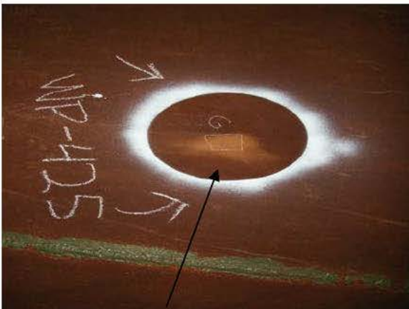
C2-P35-1 PIT REPAIR
