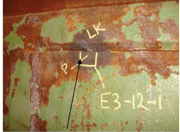
E3-P12-1 WELD REPAIR- LEAK
