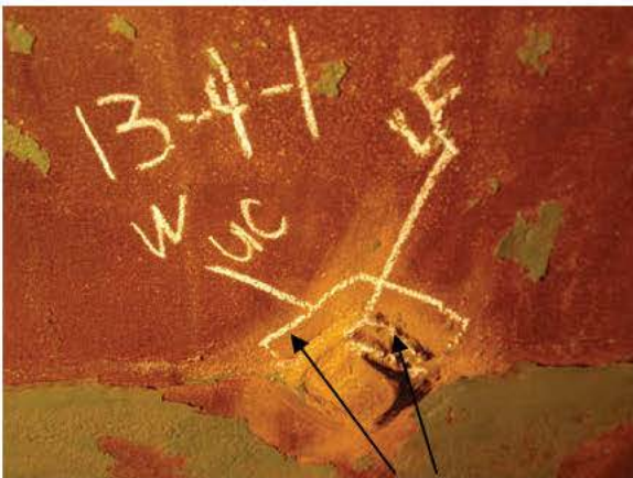
R13-P4-2 WELD REPAIR- UNDERCUT
