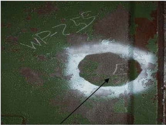
A-P5-1 PIT REPAIR
