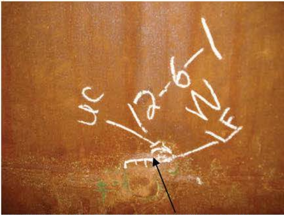
R12-P6-2 WELD REPAIR- UNDERCUT
