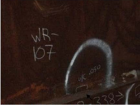
R1-P8-2 WELD REPAIR- UNDERCUT
