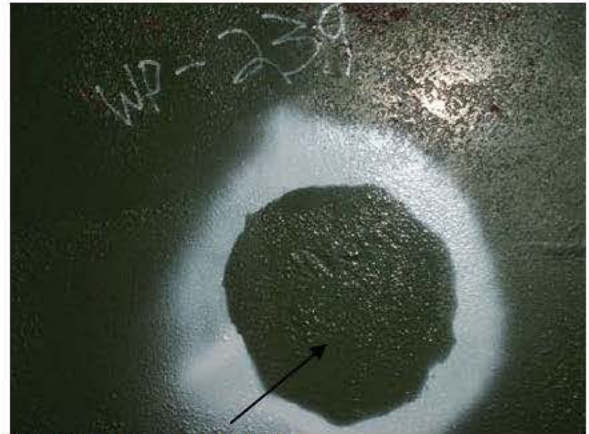
B-P30-1 PIT REPAIR
