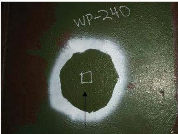
B-P27-2 PIT REPAIR
