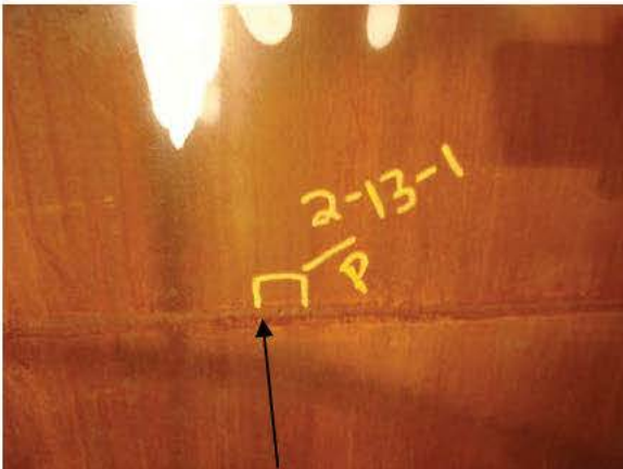
R2-P13-1 WELD REPAIR- POROSITY
