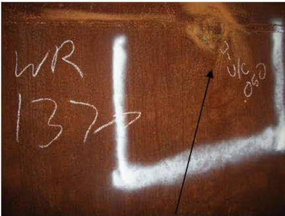
R12-P8-1 WELD REPAIR- UNDERCUT
