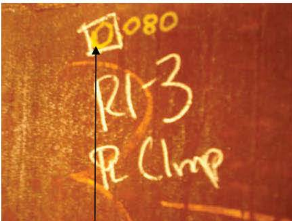
R1-P3-1 PLATE CLAMP REPAIR
