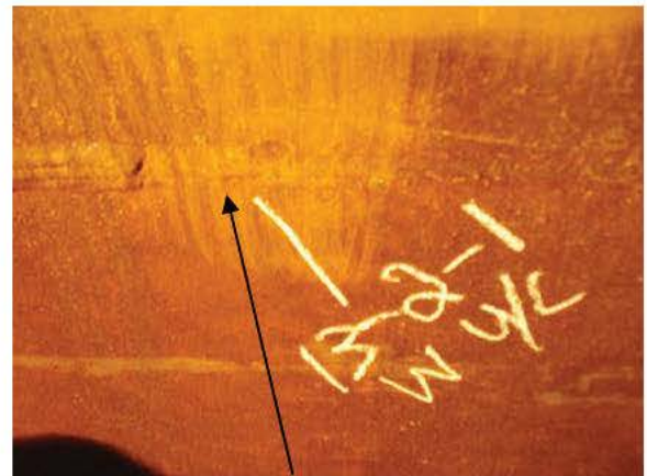
R13-P2-1 WELD REPAIR- UNDERCUT
