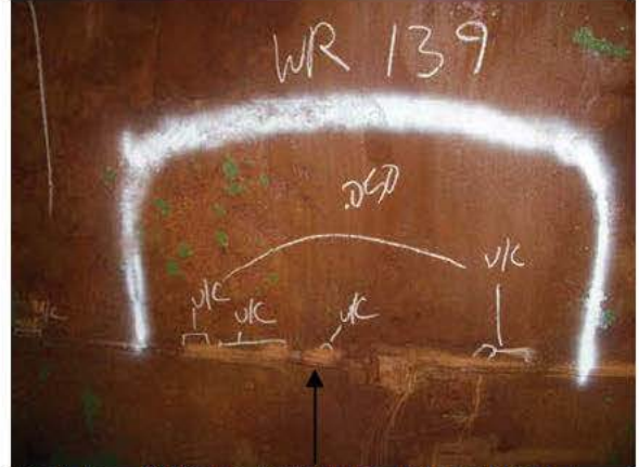
R20-P8-4 WELD REPAIR- UNDERCUT
