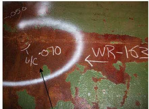
R22-P9-2 WELD REPAIR- UNDERCUT
