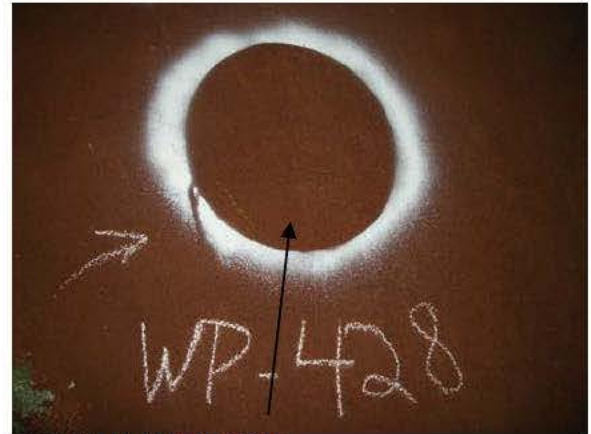
C2-64-1 PIT REPAIR
