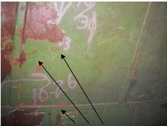
C-1-2 GOUGE & WELD REPAIR- UNDERCUT
