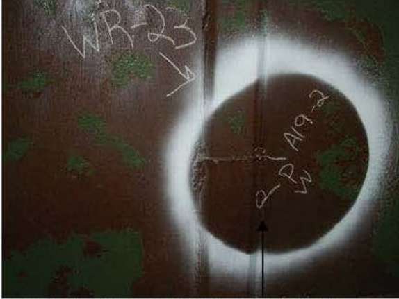
A-P19-2 WELD REPAIR- POROSITY
