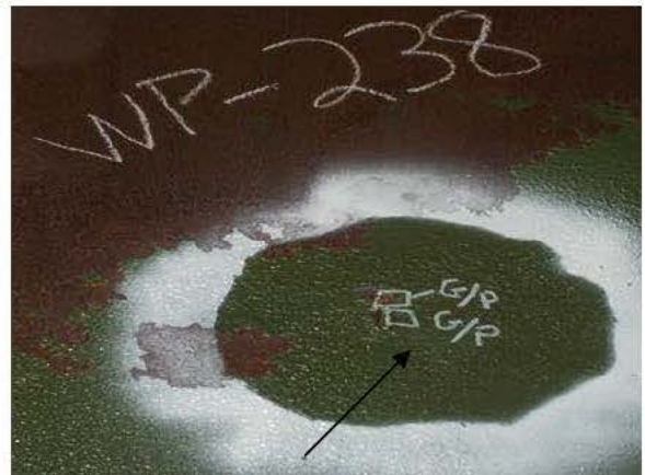
B-P36-1 PIT REPAIR
