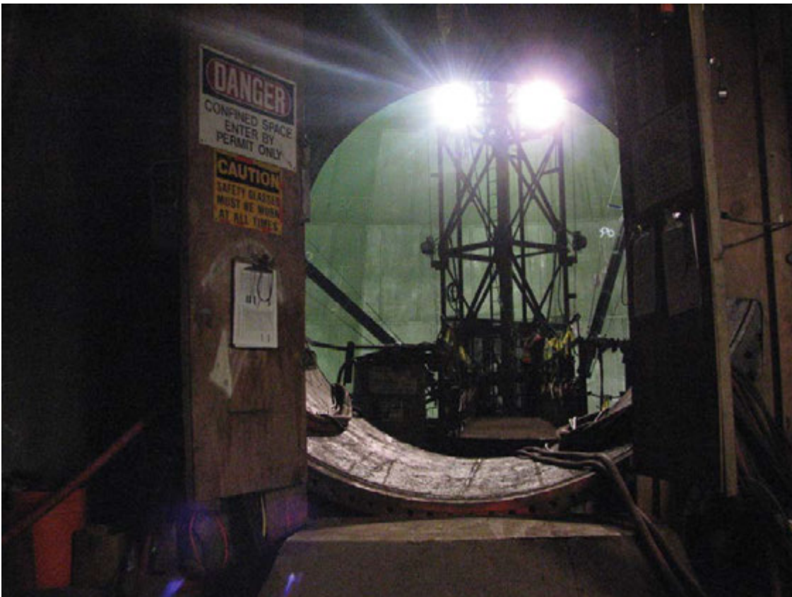
A view of the manway (Typical Tank Access)
