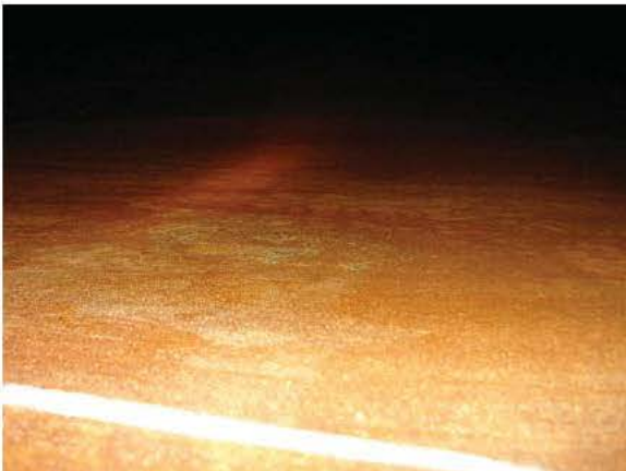
R16-1 GENERAL CONDITION
