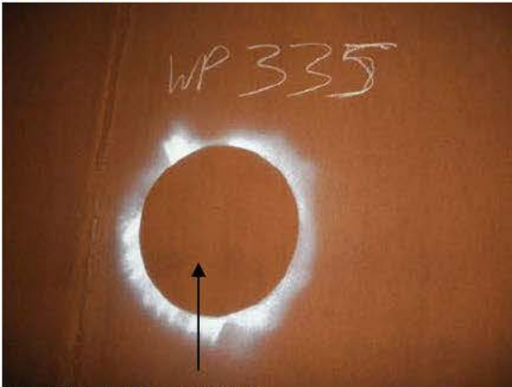
C3-P29-1 PIT REPAIR
