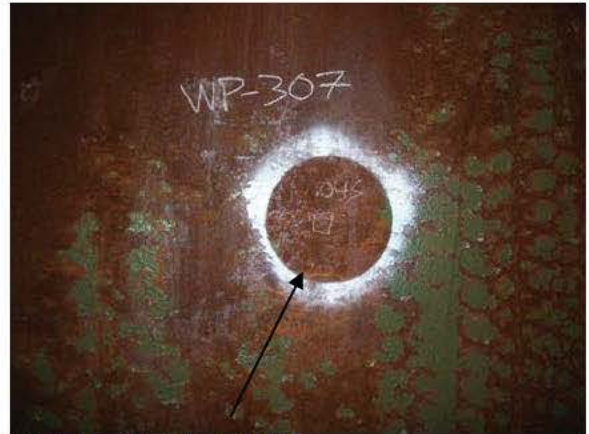
R13-P4-3 PIT REPAIR
