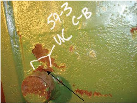
B-P59-3 WELD REPAIR- UNDERCUT
