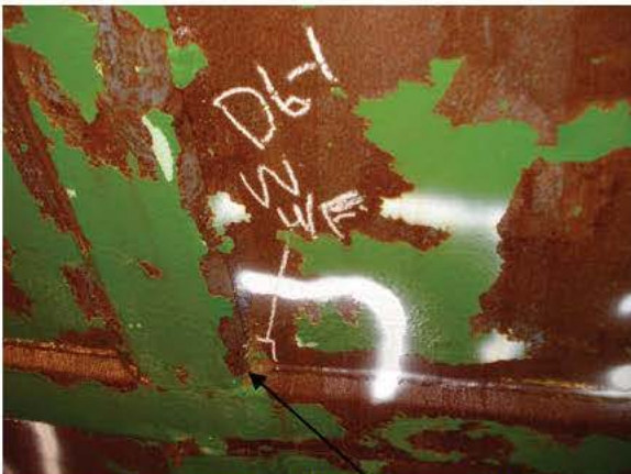
D-P6-1 WELD REPAIR- UNDERFILL
