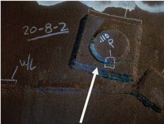
R20-P8-2 WELD REPAIR-POROSITY
