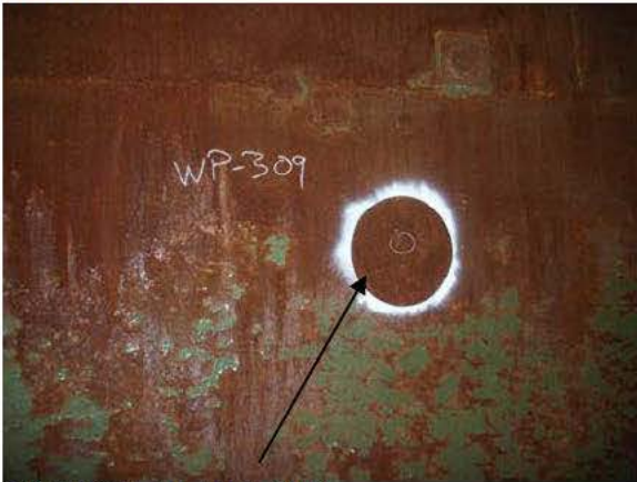
R13-P2-2 PIT REPAIR
