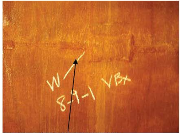
R8-P9-1 WELD UNIFORMITY
