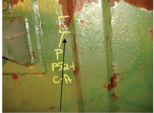
A-P52-1 PIT REPAIR
