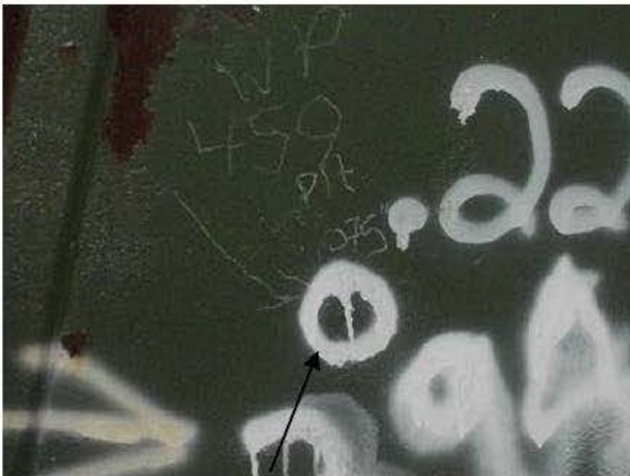
D-P25-3 PIT REPAIR
