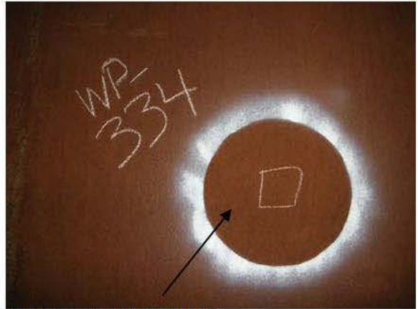
C3-P24-1 PIT REPAIR
