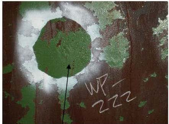
D-P16-1 PIT REPAIR
