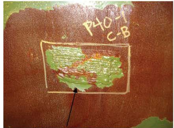
B-P40-1 WELD BUILD UP
