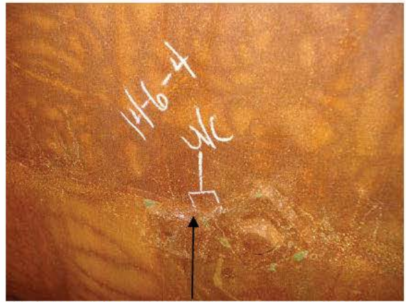
R14-P6-4 WELD REPAIR- UNDERCUT
