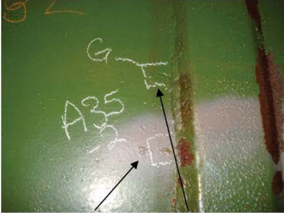
A-P35-2 PIT & GOUGE REPAIR
