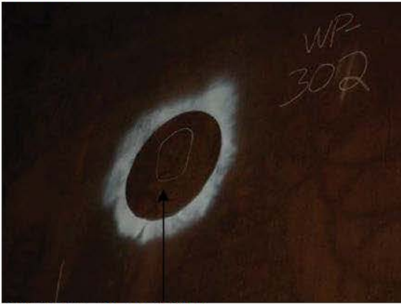
R13-P7-2 PIT REPAIR
