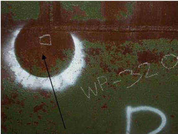
R23-P4-1 PIT REPAIR
