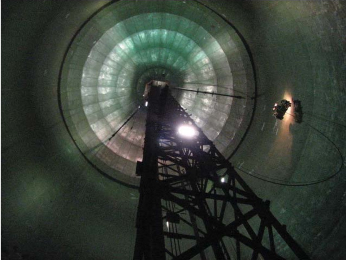
A view from the tank bottom of one of the teams scanning the barrel
