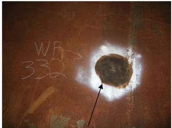
C2-P18-1 PIT REPAIR
