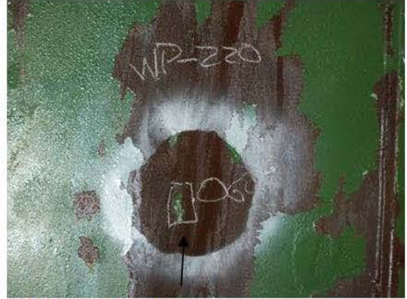
D-P19-1 PIT REPAIR
