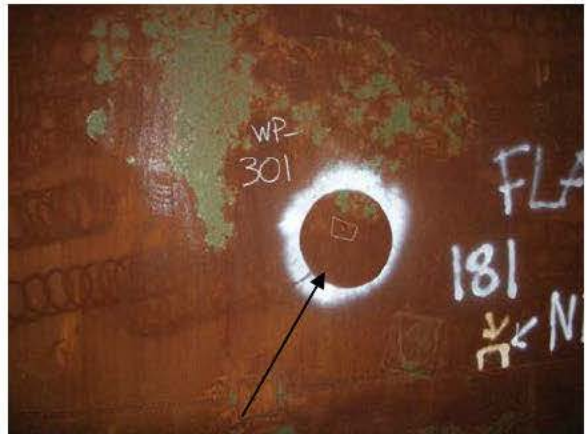
R11-P6-3 PIT REPAIR
