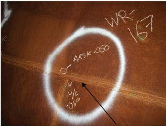
R11-P8-1 WELD REPAIR- UNDERCUT
