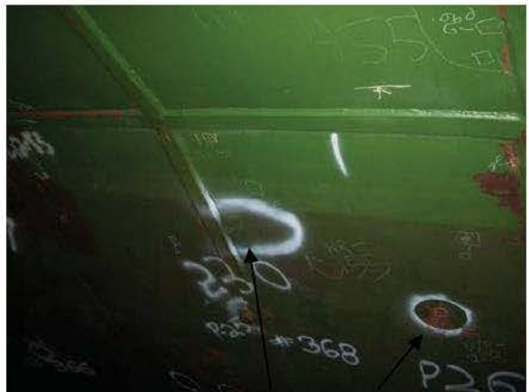
C-P26-1 GOUGE & WELD REPAIR- UNDERCUT
