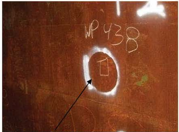
R9-P1-1 PIT REPAIR
