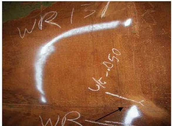
R10-P8-1 WELD REPAIR- UNDERCUT
