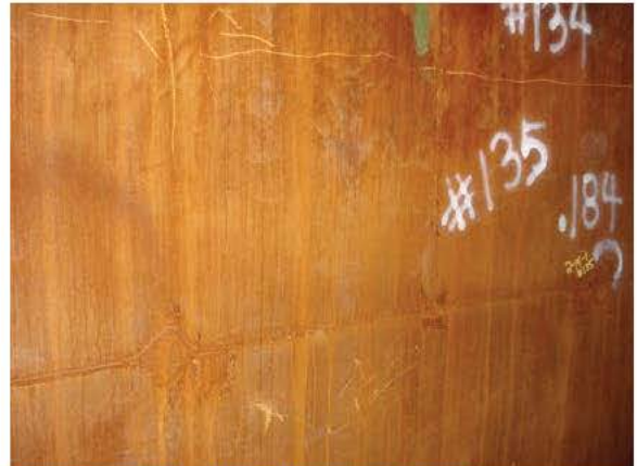
R2-P14-3 GENERAL CONDITION
