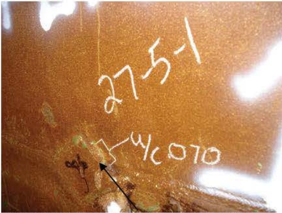
R27-P5-1 WELD REPAIR- UNDERCUT
