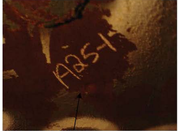
A-P25-1 PIT REPAIR
