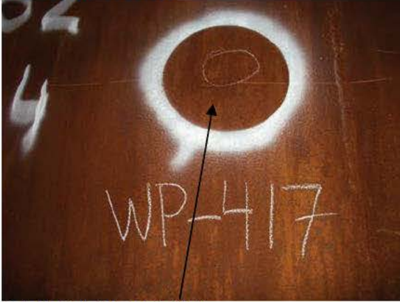
C4-P52-1 PIT REPAIR
