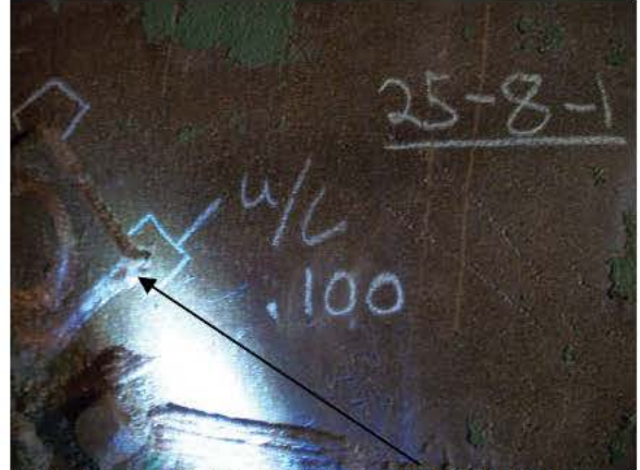
R25-P8-1 WELD REPAIR- UNDERCUT
