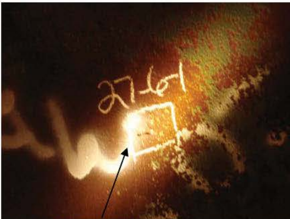
R27-P6-1 PIT REPAIR
