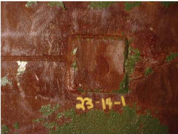
R23-P14-1 GENERAL CONDITION
