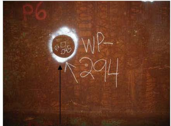
R6-P6-1 PIT REPAIR
