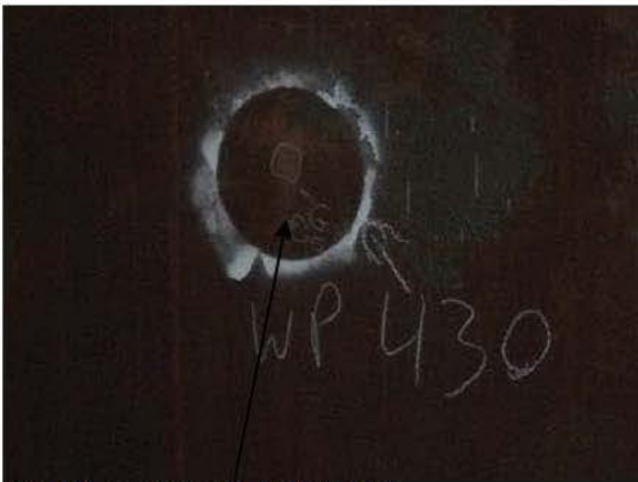
C3-P1-2 GOUGE REPAIR
