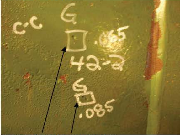
C-P42-2 GOUGE REPAIRS
