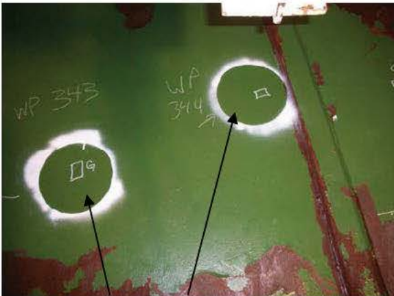
D-P32-1 GOUGE REPAIRS
