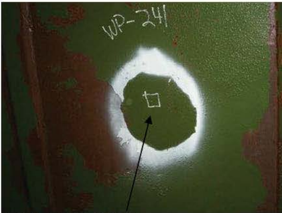
B-P27-1 PIT REPAIR
