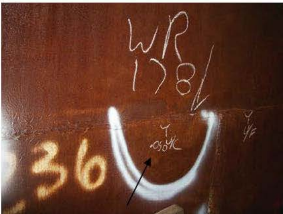
R10-P16-1 WELD REPAIR- UNDERCUT
