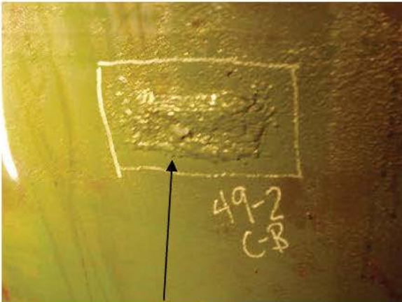
B-P49-2 WELD BUILD UP
