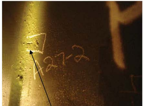
A-P27-2 PIT REPAIR
