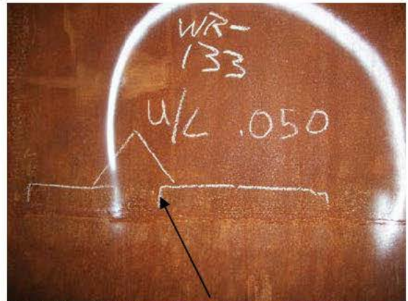
R11-P8-4 WELD REPAIR- UNDERCUT
