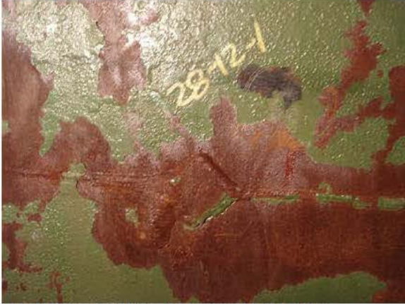
R28-P12-1 GENERAL CONDITION
