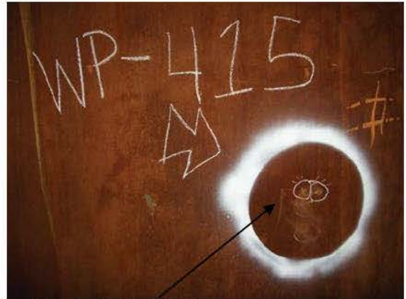
R5-P9-1 PIT REPAIR
