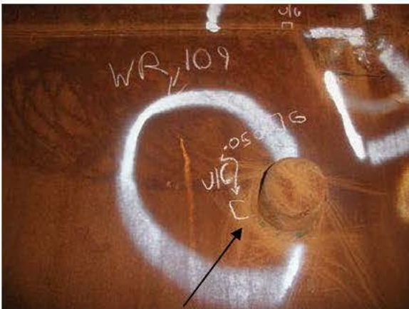
R5-P8-2 WELD REPAIR- UNDERCUT
