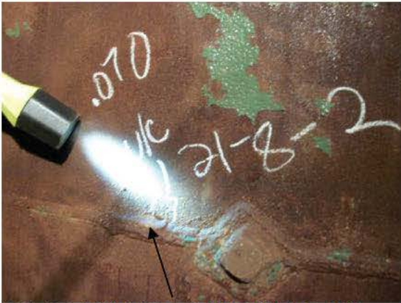
R21-P8-2 WELD REPAIR- UNDERCUT
