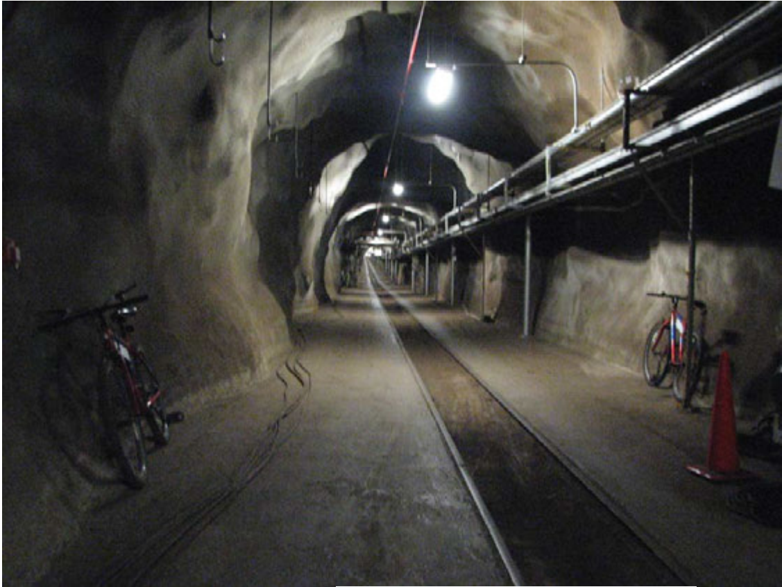
A view of the tunnel area around tank
