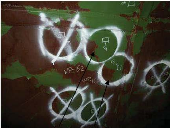
C-P38-2 GOUGE REPAIRS
