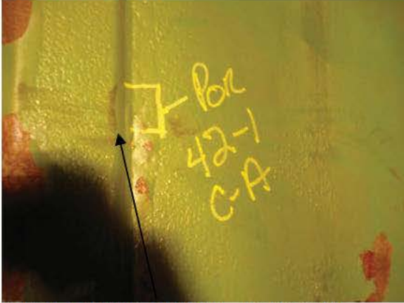
A-P42-1 WELD REPAIR- POROSITY
