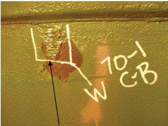
B-P70-1 WELD BUILD UP
