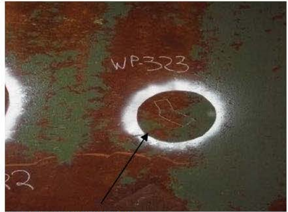
R24-5-2 PIT REPAIR
