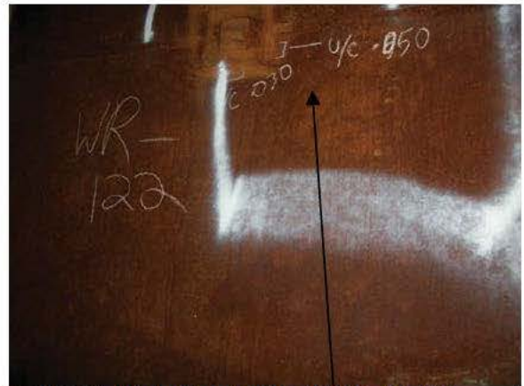
R6-P8-2 WELD REPAIR- UNDERCUT
