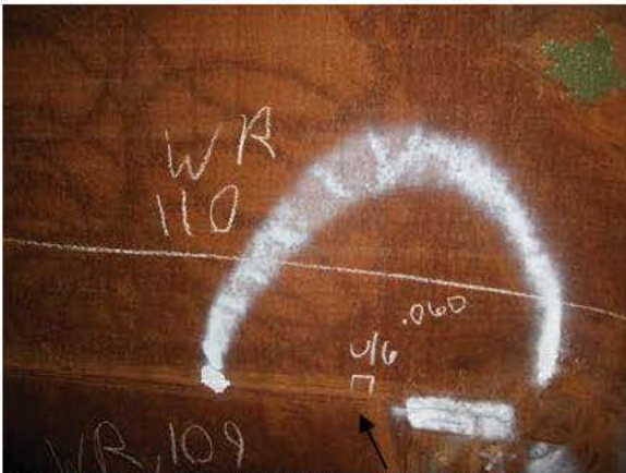
R6-P9-1 WELD REPAIR- UNDERCUT
