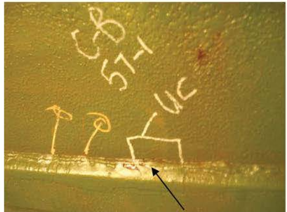
B-P57-1 WELD REPAIR- UNDERCUT
