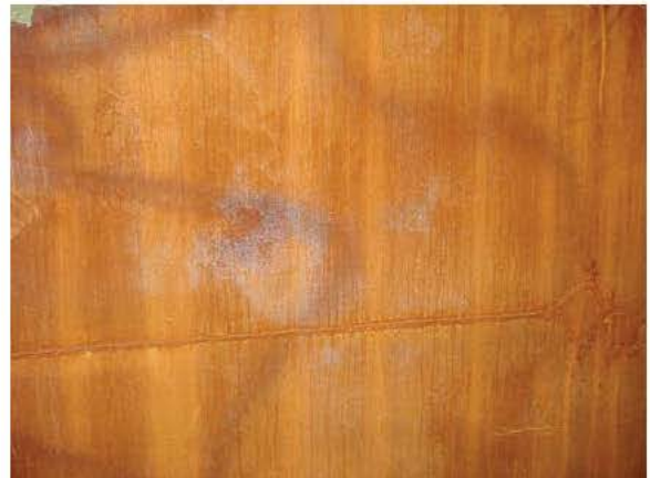
R2-P14-4 GENERAL CONDITION
