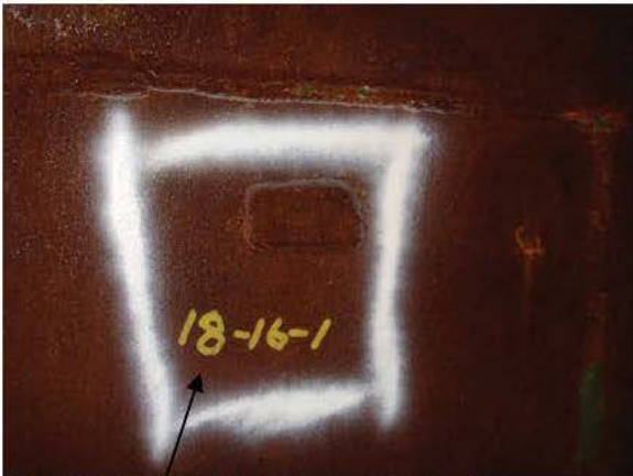
R18-P16-1 GENERAL CONDITION
