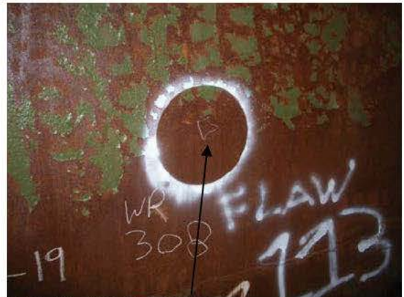
R13-P4-4 PIT REPAIR
