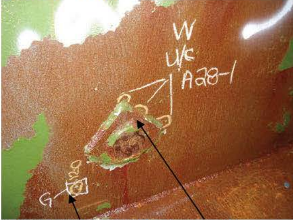
A-P28-1 GOUGE & WELD REPAIR- UNDERCUT
