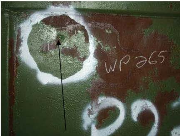
A-P23-1 PIT REPAIR
