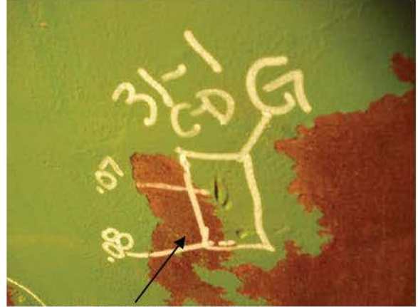
D-P31-1 GOUGE REPAIRS
