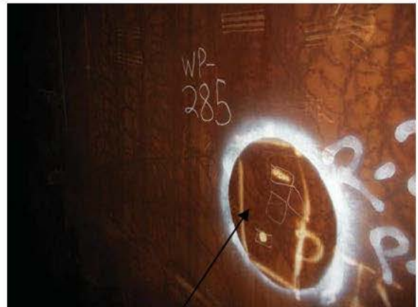
R2-P8-2 PIT REPAIRS
