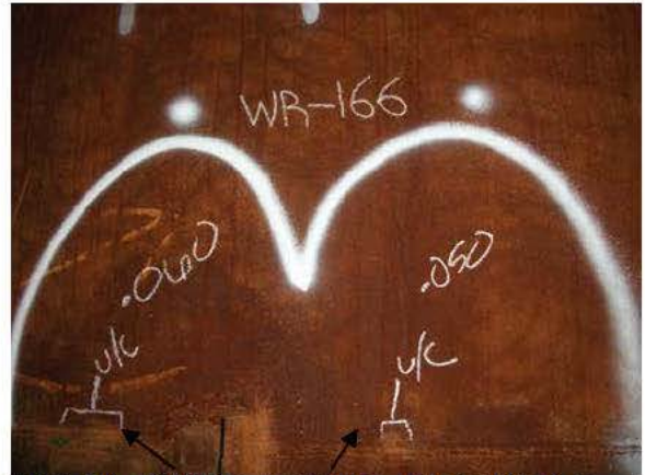
R12-P9-1 WELD REPAIR- UNDERCUTS
