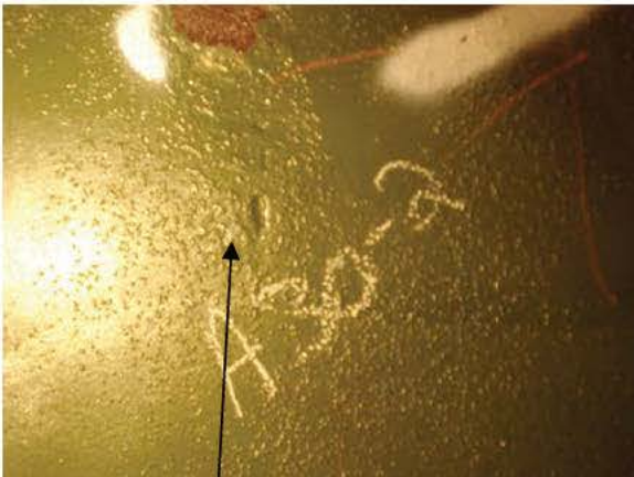
A-P30-2 PIT REPAIR
