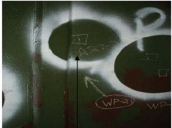
A-26-1 PIT REPAIR
