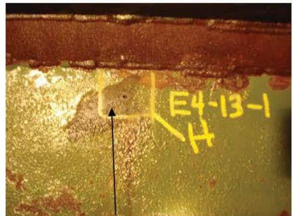
E4-P13-1 HOLE REPAIR
