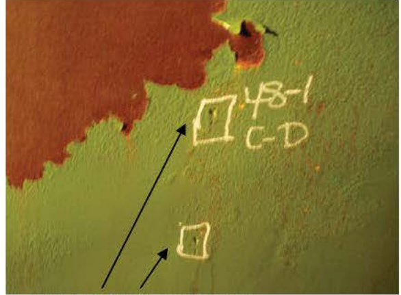
D-P48-1 GOUGE REPAIRS
