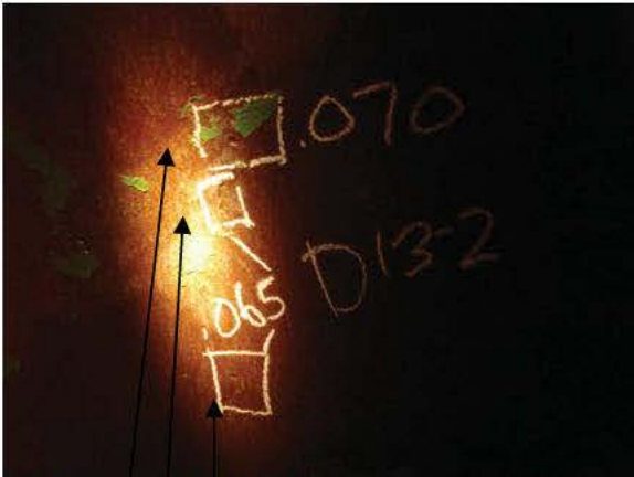
D-P13-2 GOUGE REPAIRS
