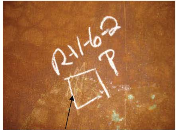
R11-P6-2 PIT REPAIR
