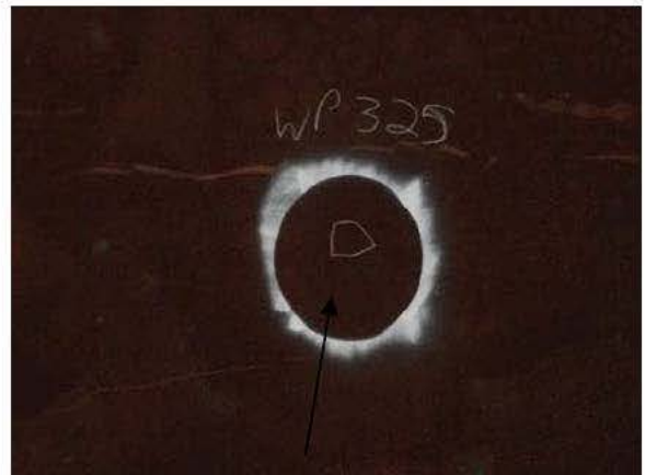
R24-P7-2 PIT REPAIR
