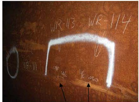
R6-P8-1 WELD REPAIR- UNDERCUT
