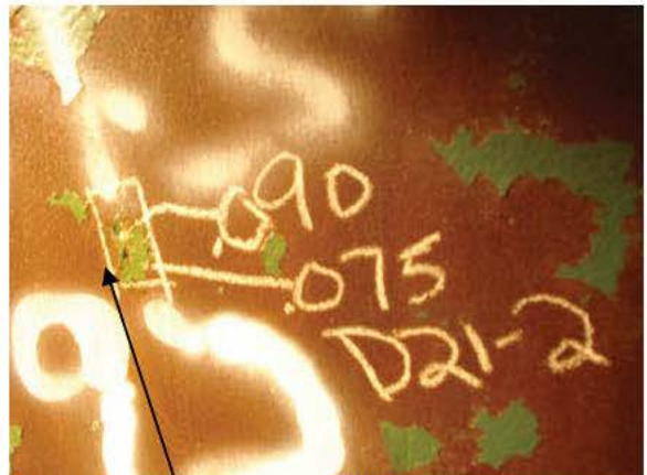
D-P21-2 GOUGE REPAIRS
