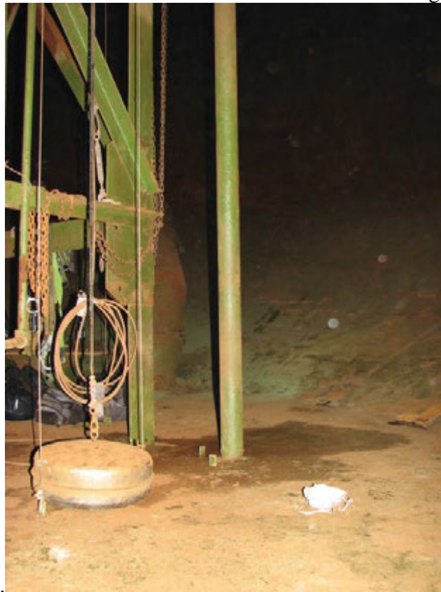
Picture showing part of the floor and lower dome
