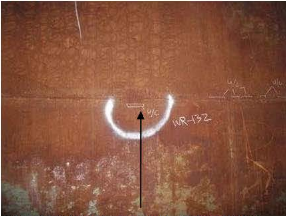
R11-P7-1 WELD REPAIR- UNDERCUT
