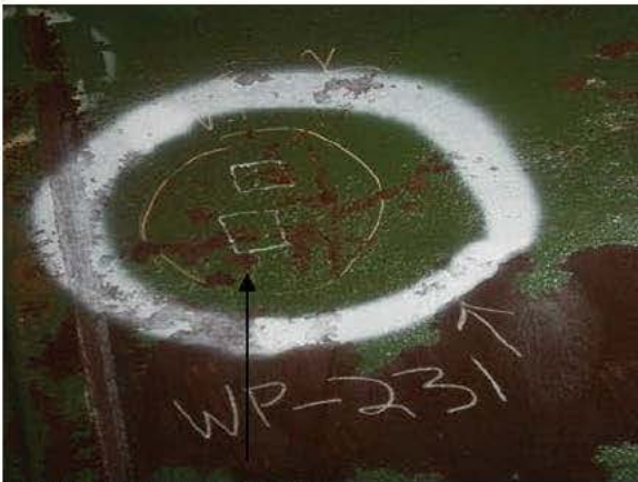
C-P16-2 PIT REPAIRS
