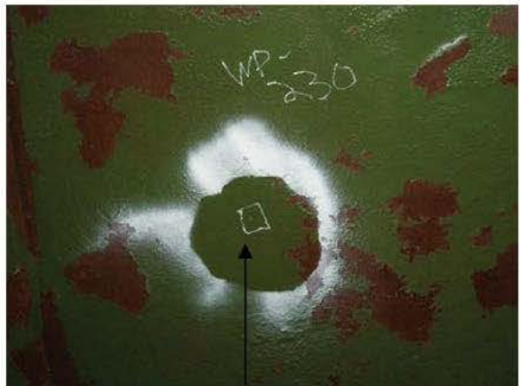
C-P11-1 PIT REPAIR
