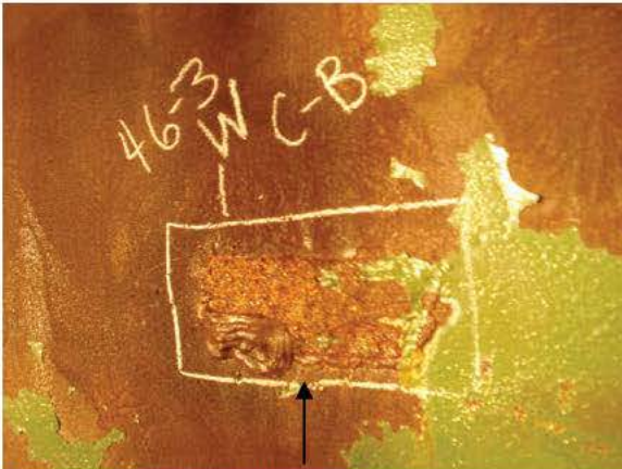
B-P46-3 WELD BUILD UP
