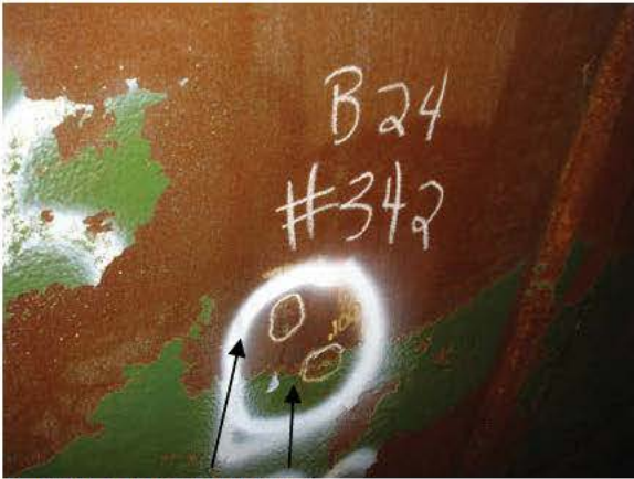
B-P24-1 PIT REPAIR
