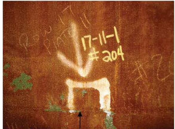
R17-P11-1 WELD REPAIR- UNDERCUT
