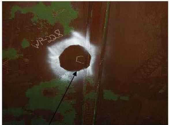
C-P8-1 PIT REPAIR
