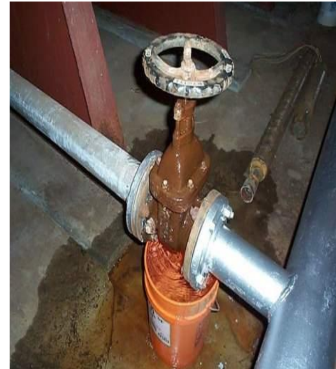
Leaking valve
