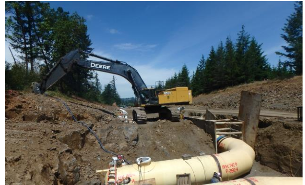
Willamette Water Supply System Pipeline Construction
