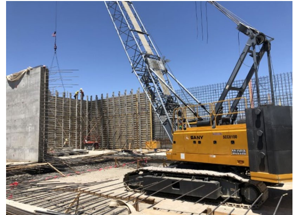
Aeration Basin Construction
