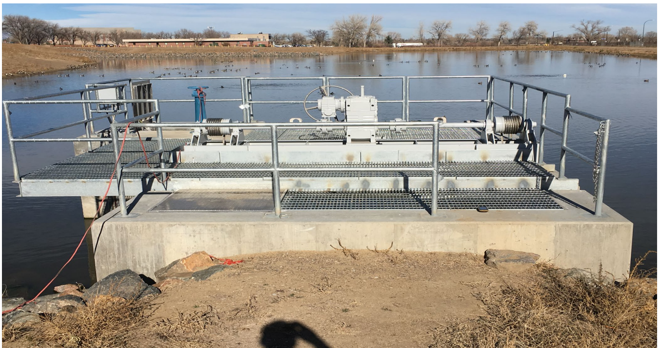
Figure 5 – Downing Reservoir Outlet Structure
