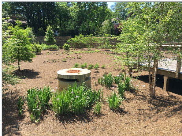
Figure 2. The bioretention area filters and treats the first flush of urban stormwater runoff.
