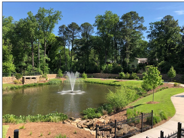
Figure 3. The main pool provides storage volume for water quality/channel protection and outlet control.
