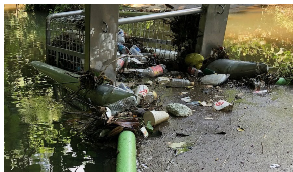
Trash catchment system at Proctor Creek.
