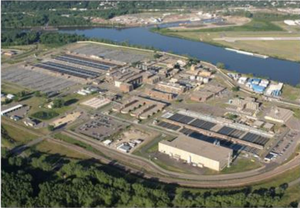
Metropolitan Wastewater Plant, St. Paul
