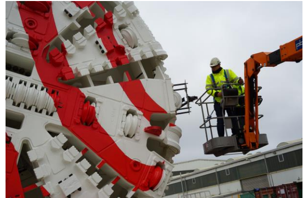
King County Ship Canal Construction
