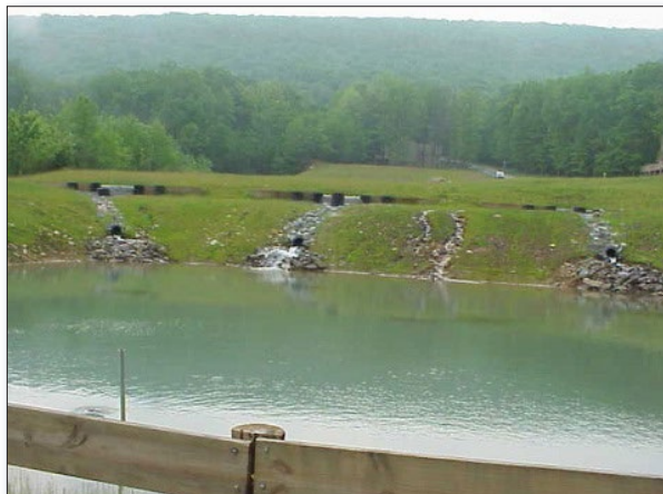
Figure 2. The Oneida #1 treatment system discharges through oxalic limestone drains into a settling pond.
