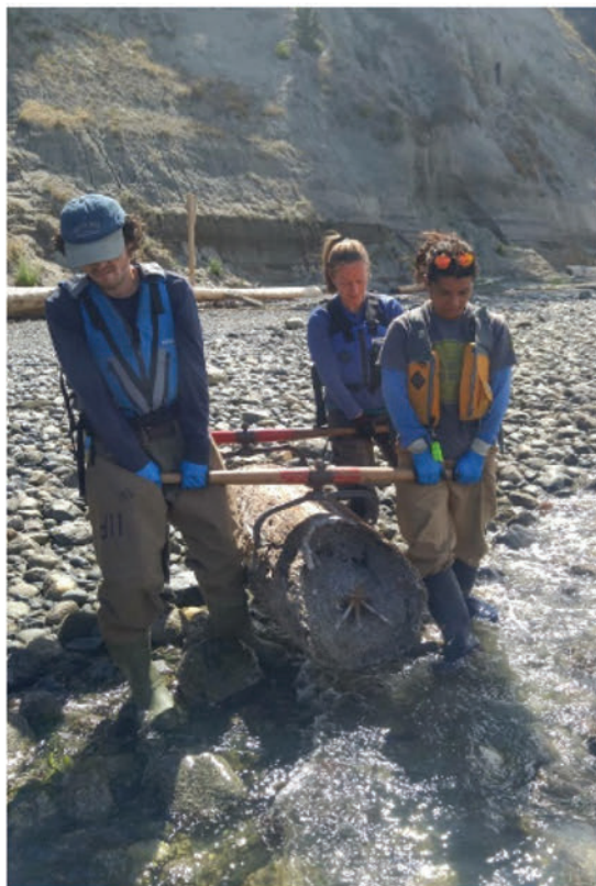
A creosote piling being removed from Lopez Island, WA.
