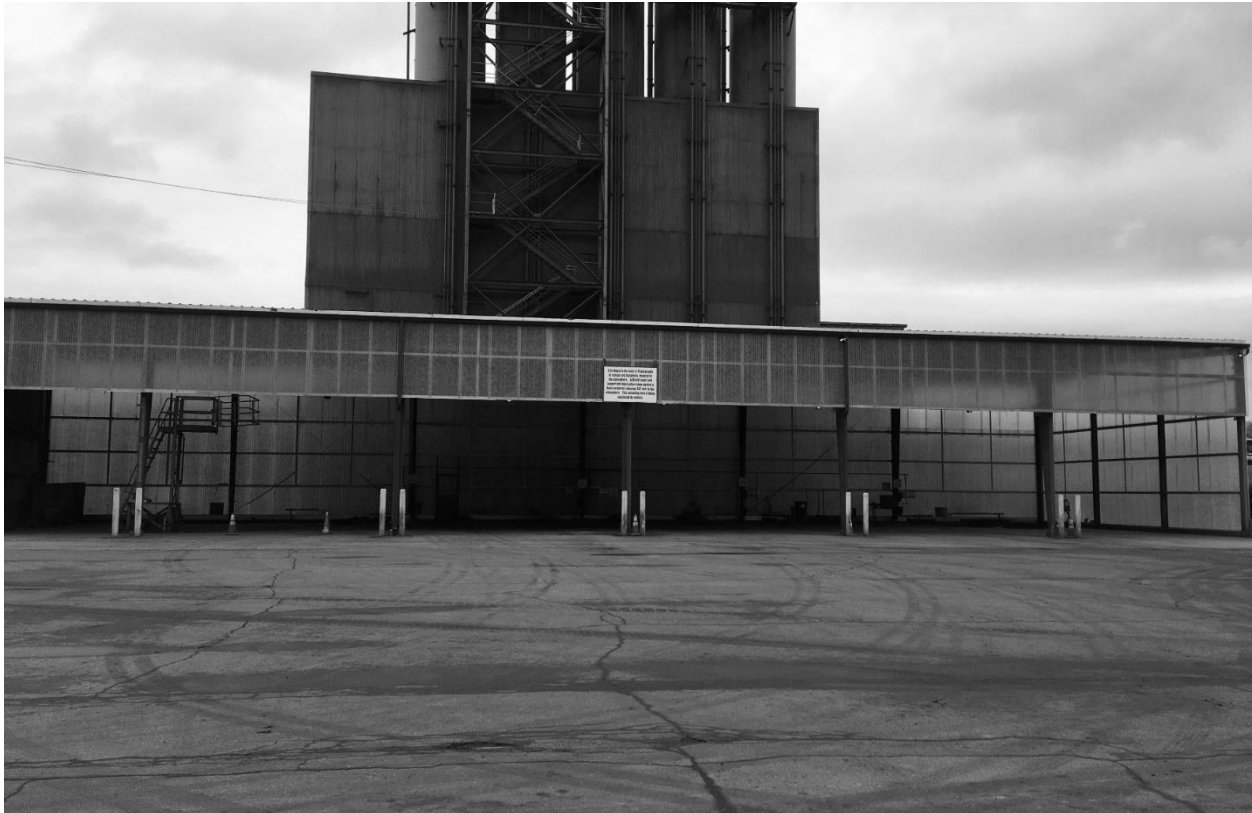
Figure 3 – Example Pneumatic Unloading (EAF PD Unloading Area)
