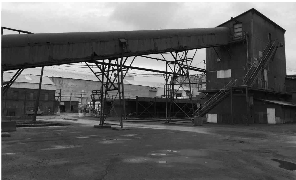
Figure 1 - Example Roadway Area
