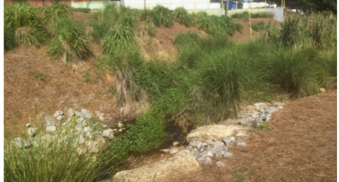
Mr. Tucker shared photographs of green infrastructure with the class that he spotted along White Street in the West End community. He noted, “the bioswales are situated in a manner to catch rainwater runoff from huge parking lots on the hill above them.”
