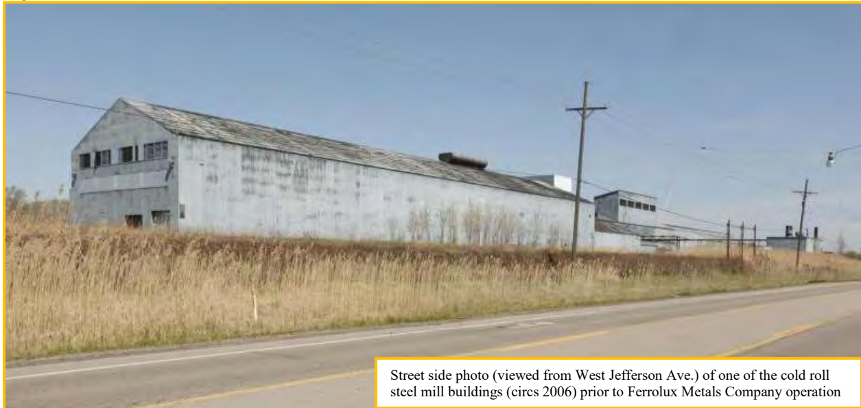
Figure 7 – McLouth Gibraltar Cold Roll Steel Mill
