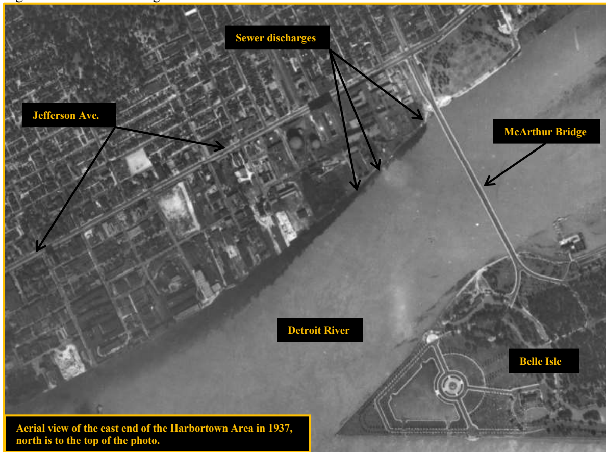
Figure 8 – Sewer discharge into the Detroit River
