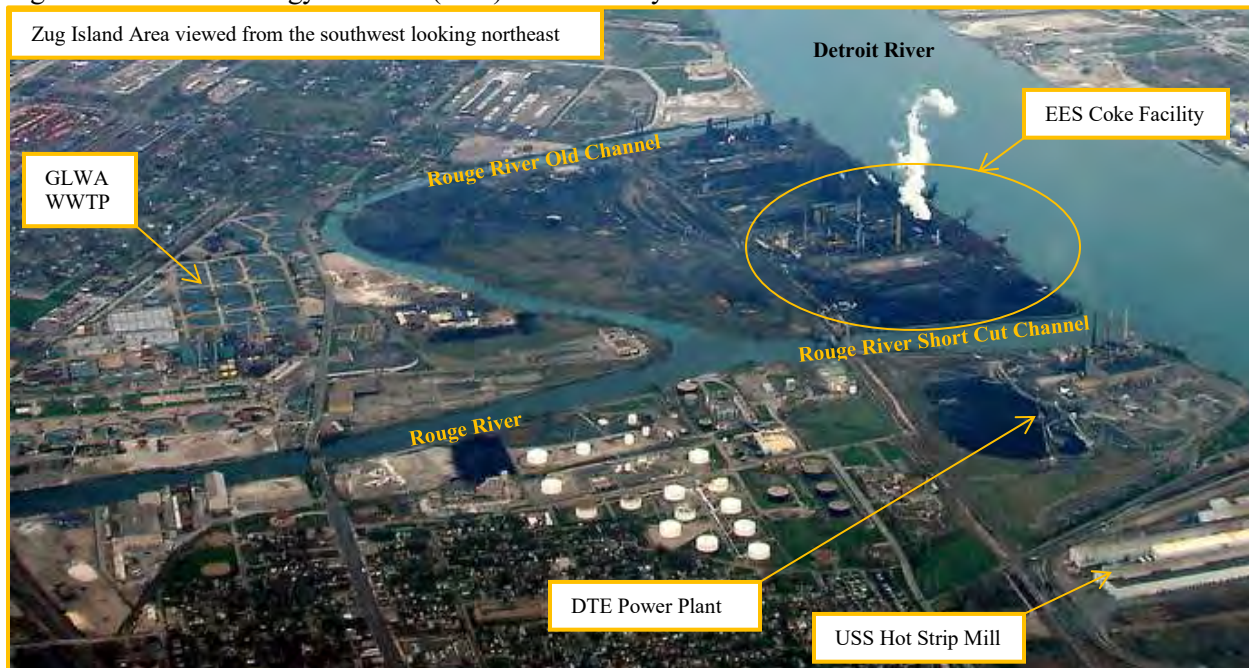
Figure 13 - Edison Energy Services (EES) Coke Battery
