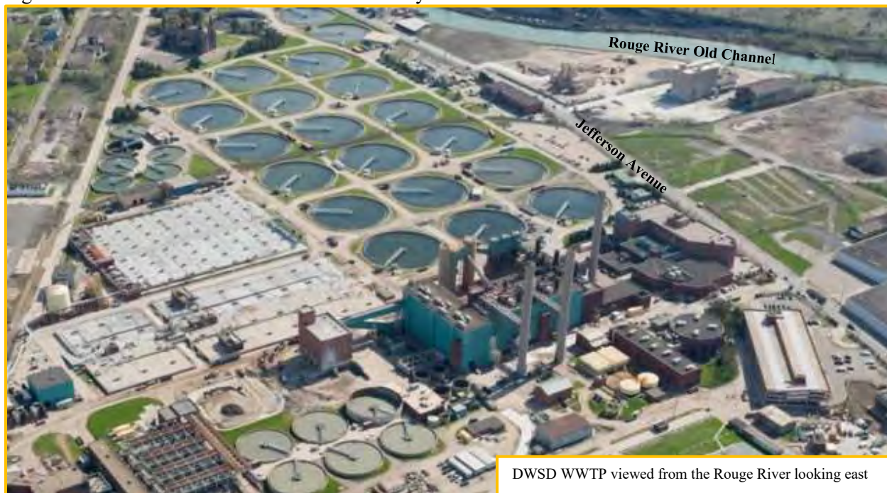
Figure 21 – Detroit Waste Water treatment facility
