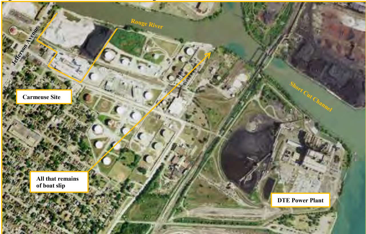
Figure 18 – 2016 Aerial Photo of Lower Rouge River and Short Cut Channel
