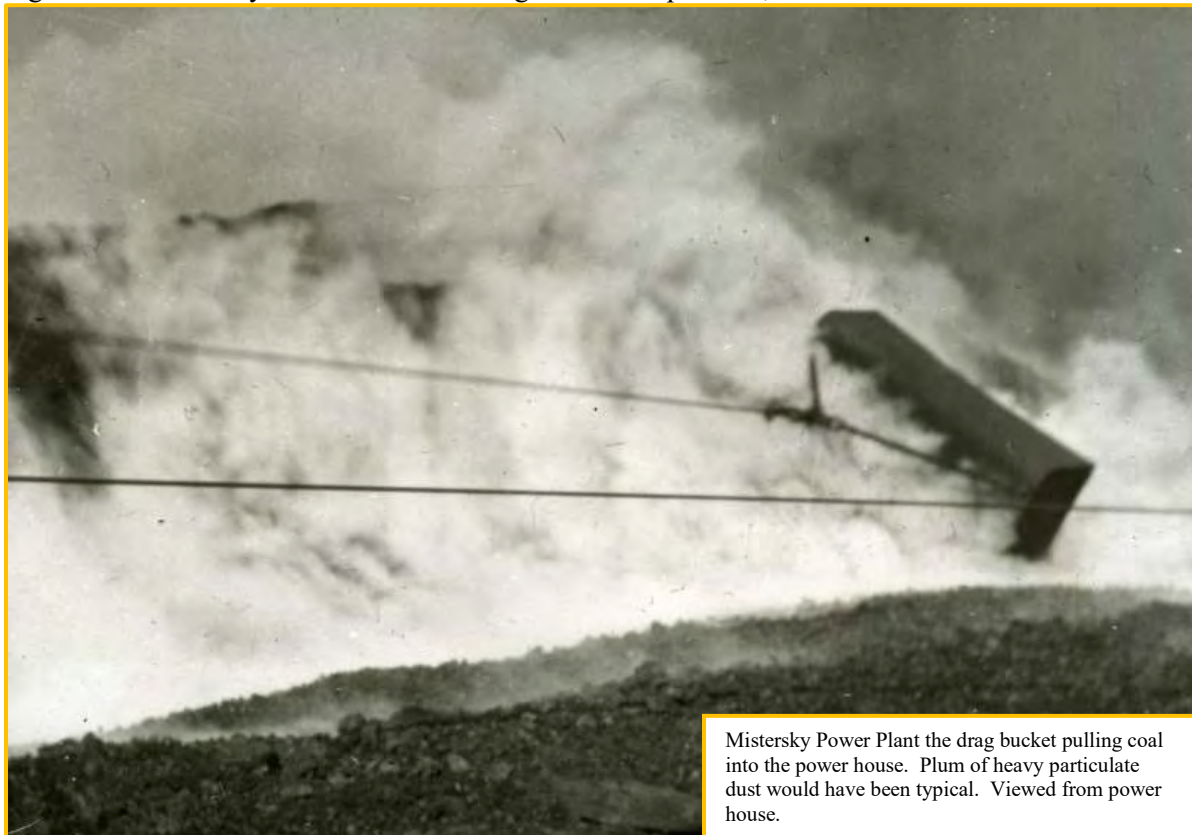
Figure 17 – Mistersky Power Plant coal drag bucket in operation, circa 1928
