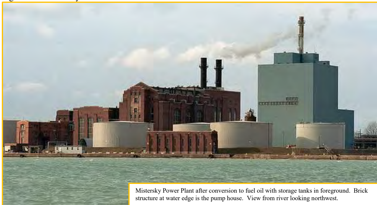
Figure 14 – Mistersky Power Plant
