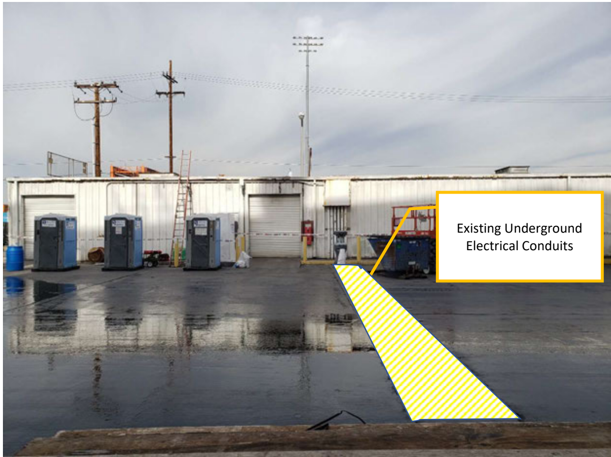
Photograph 2: BESS Building (Facing North)
