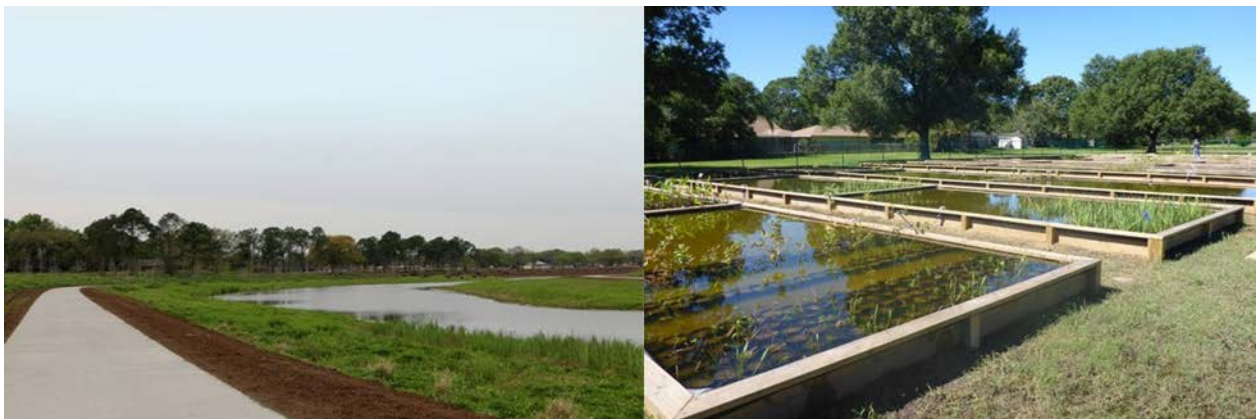
Photos above from the Exploration Green project in Texas where the Galveston Bay Estuary Program partnered in converting a former golf course of 178-acres into a large park to help manage stormwater, reduce flooding hazards, and protect regional water supplies. Photo on left of stormwater basin/pond created and photo on right of wetland nursery. (Source: Galveston Bay Estuary Program).
