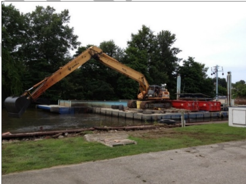
Figure 4: Dredging at Jack's Marine North Slip
